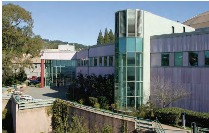
North side of the Advanced Light Source Facility
