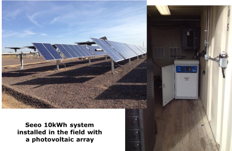
Figure 18: Field Installation of Seeo 10 kWh Energy Storage System
