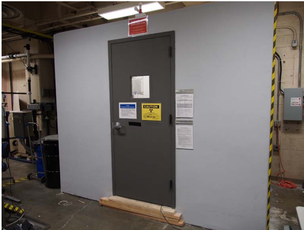
Figure 1-8. External view of the X-PREX shielding enclosure.
