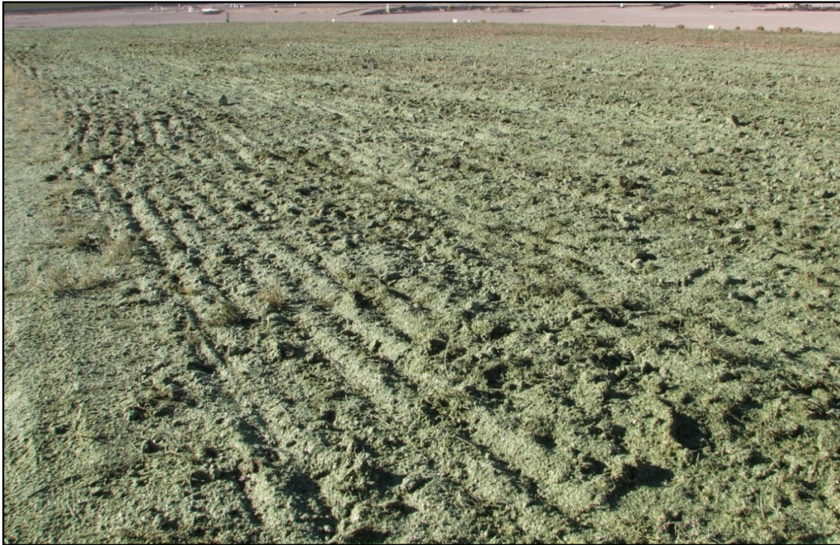
Figure 7-2. Hydromulch application on the North-North Cover, October 2013
