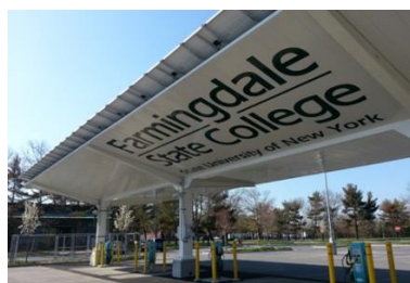
(a) Solar Carport
