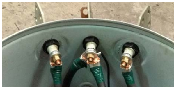
Figure 3.7. Connection of the LV leads to the bushing terminals.
