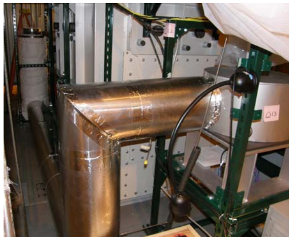
Figure 74 – External Loop with Metal Cladding
