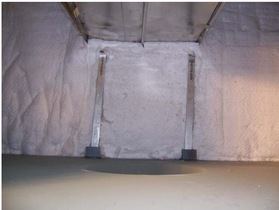
Figure 25 – Peripheral Insulation Blankets at Mid-elevation (fuel inlet side)
