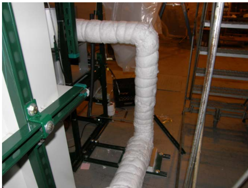
Figure 31 – Recirculation Loop Piping Insulation in Progress
