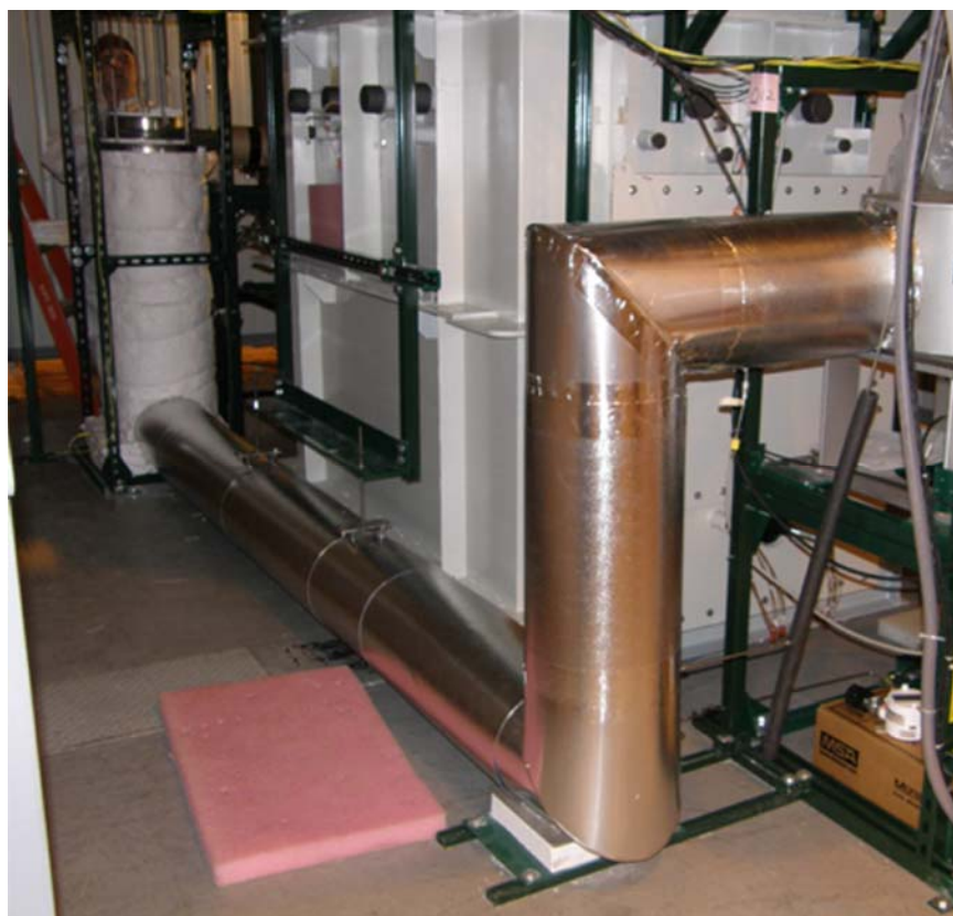
Figure 32 – Finished Recirculation Loop Pipe between Circulator and Fuel Heater No. 1
