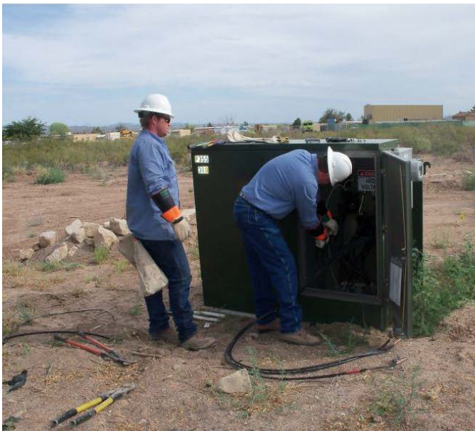
Connecting System to the Grid
