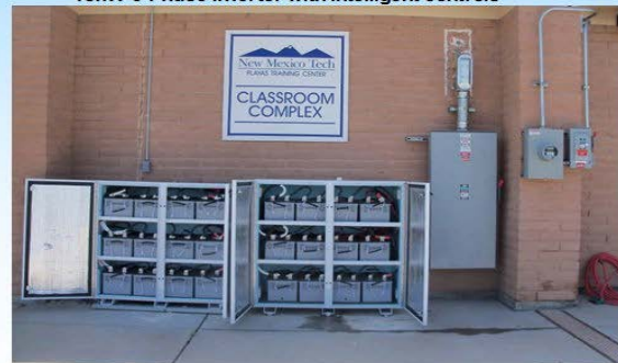
72kWhrs of Battery Backup
