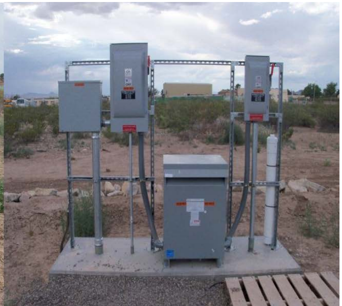
Visible Grid Connect/Disconnect
