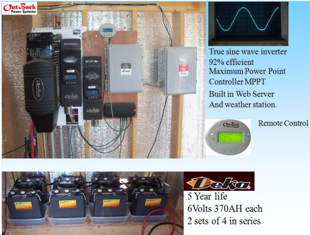
Figure 12. Laguna 12 Inverter and Batteries
