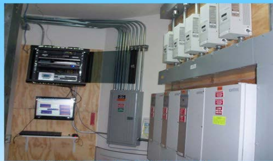
18kW 3-Phase Inverter with Intelligent controls
