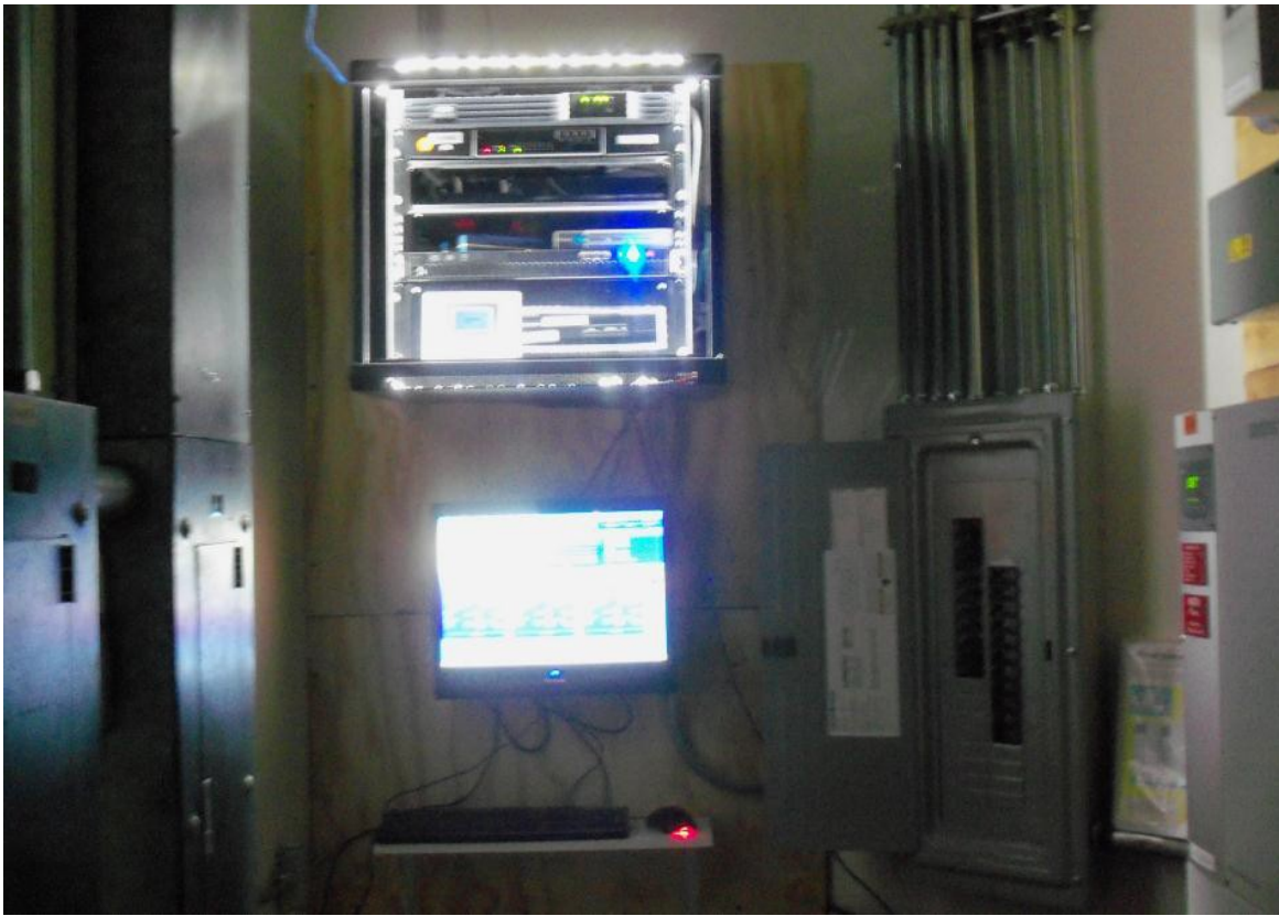
Figure 29. IT Platform Running During Total Grid Failure
