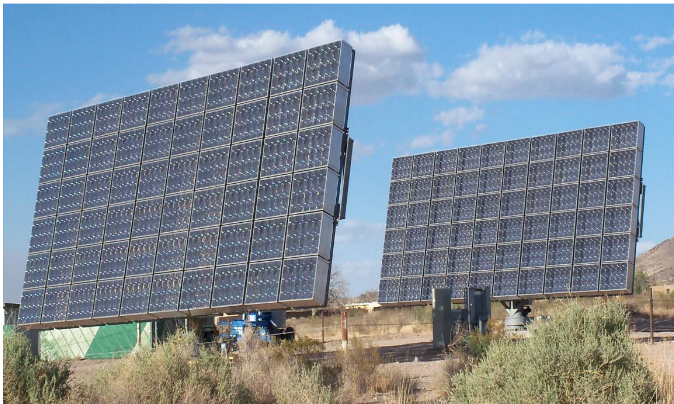
Figure 14. 50 kW Grid-Connected EMCORE PV System
