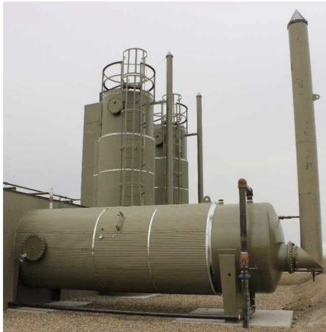
Figure 3-11. Installed Horizontal and Vertical HTs.
