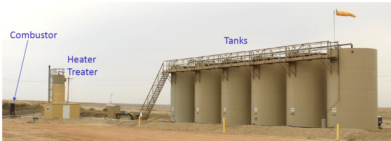
Figure 3-7. Bakken Well Site Conditioning Equipment Configuration.
