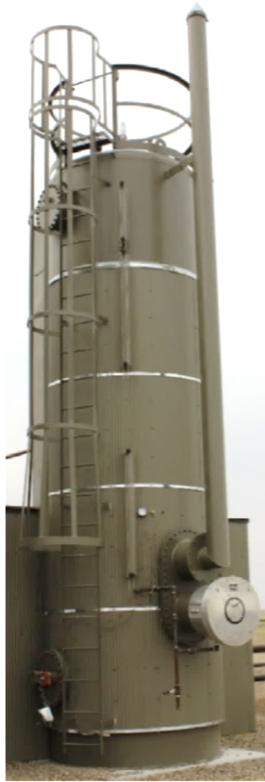
Figure 3-10. Installed Vertical HT.
