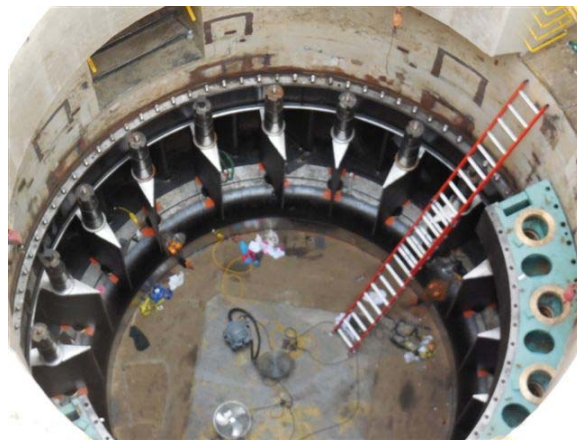
Fig. 20. Refurbished Wicket Set in Bottom Ring
