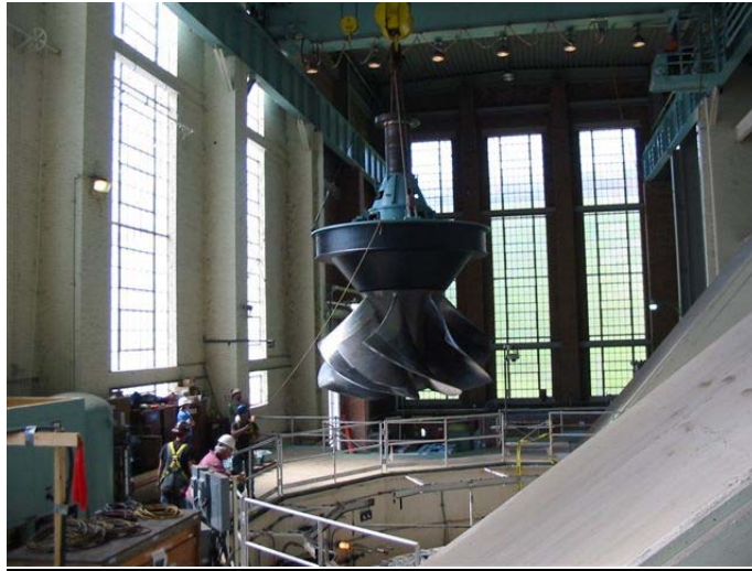
Fig. 5. Installation of Turbine, Inner Head Cover, and Bearing Housing
