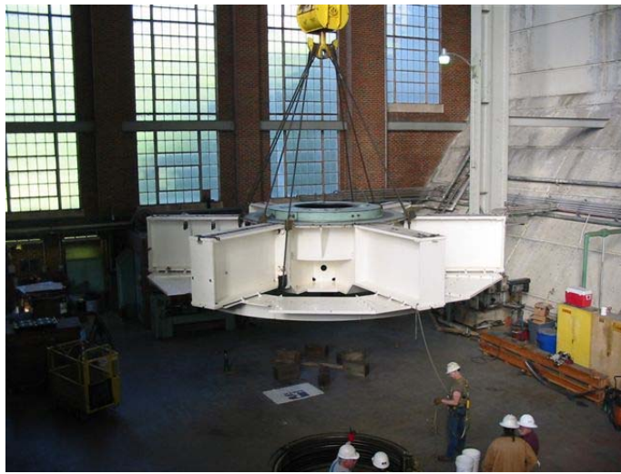
Fig. 7. Upper Bearing Bridge Installation
