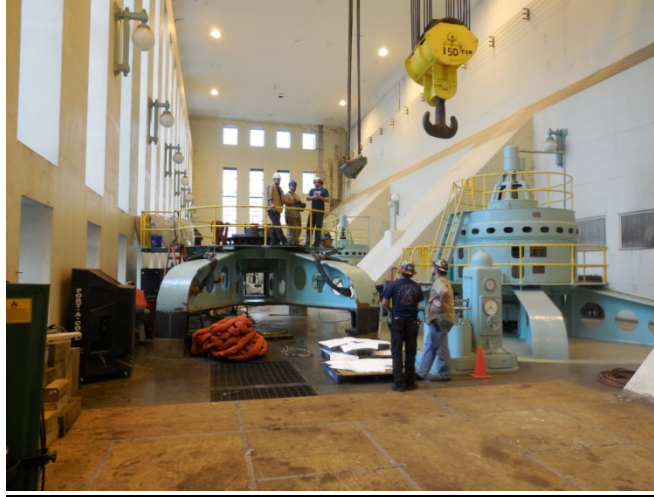
Fig. 14. Installation of New Turbine
