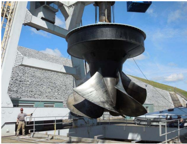
Fig. 22. Installation of New Turbine
