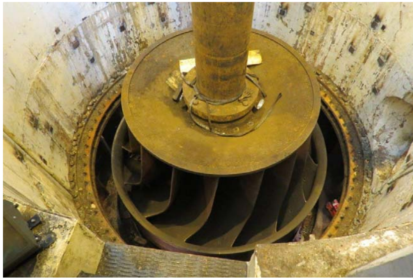
Fig. 10. Old Turbine Being Removed
