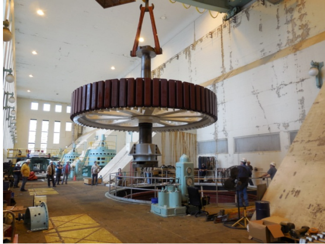
Fig. 15. Installation of Generator Rotor
