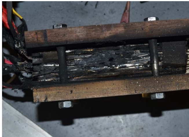
Figure 16. Photograph of the 5S1P battery post-propagation test initiated at the center cell (Cell 3).
