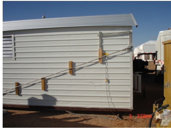
Figure H-9. Discharge relief valve.
