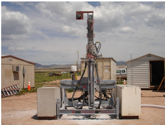
Figure H-3a. Drill rig.
