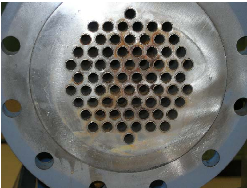
Figure 3-23: View of the Basco/Whitlock shell and tube heat exchanger gas inlet flange, showing the stainless steel tubes.
