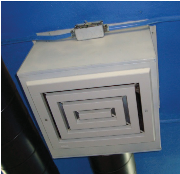
Figure 27: Faulty men's shower exhaust fan.
