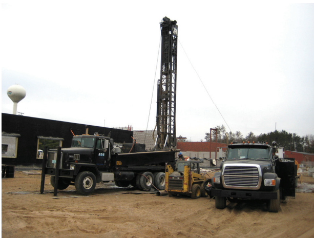
Figure 48. A typical vertical loop geothermal bore drilling operation (left) at a 54,000 ft 2 elementary school in Mosinee, WI. Figure 49. A typical vertical loop geothermal field circuit trench (right). Each vertical loop bore is located where each pair of pipes branches off and elbows down into the soil (indicated by arrow). This geothermal field serves a 113,000 ft 2 elementary school in Shawano, WI.
