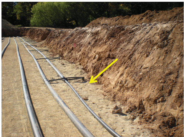
Figure 48. A typical vertical loop geothermal bore drilling operation (left) at a 54,000 ft 2 elementary school in Mosinee, WI. Figure 49. A typical vertical loop geothermal field circuit trench (right). Each vertical loop bore is located where each pair of pipes branches off and elbows down into the soil (indicated by arrow). This geothermal field serves a 113,000 ft 2 elementary school in Shawano, WI.
