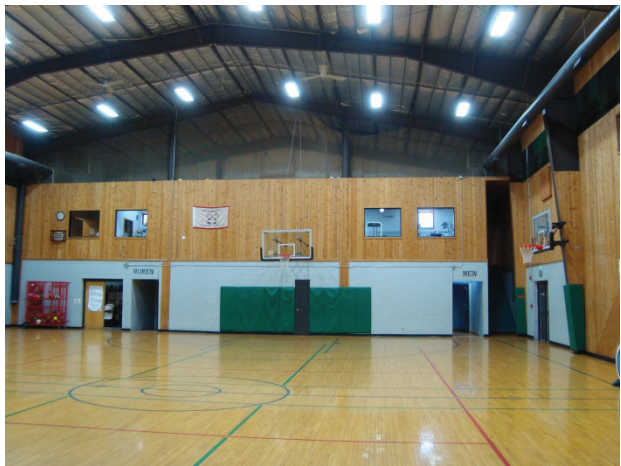
Figure 60. A view of the roof structure (right). The main beams and purlins can be seen in this photo.
