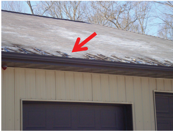
Figure 27. Heat trace heating but there is no risk of ice damming.
