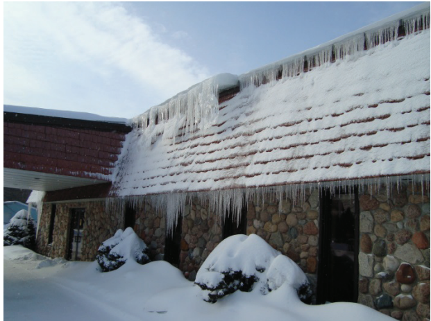
Figure 66. An example of a large sheet of ice beginning to shed off the roof (right). Sliding snow and ice should be considered as part of the structural analysis for a solar thermal system.
