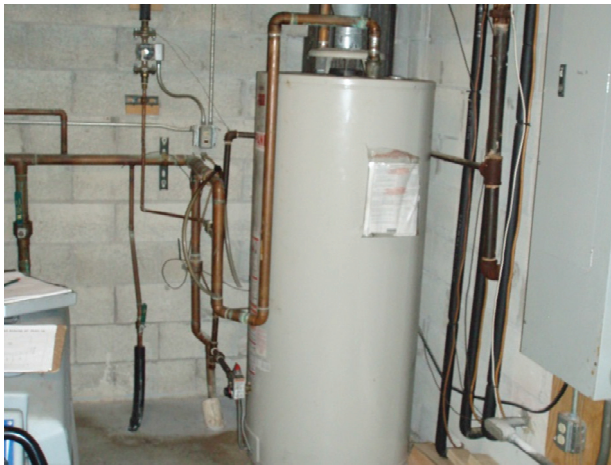
Figure 69. The domestic water heater (left).
