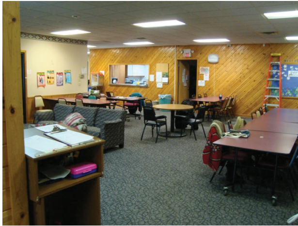
Figure 33. Typical 2' x 4' 4-lamp T8 fluorescent lighting throughout the interior (left).
