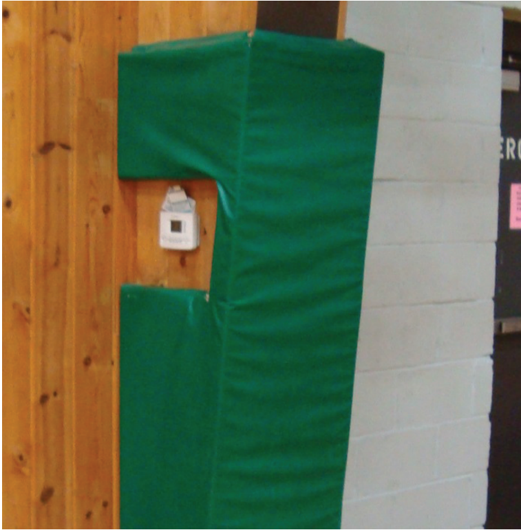
Figure 29: West gym thermostat location leading to poor temperature control and excessive furnace run time (after east unit is repaired).
