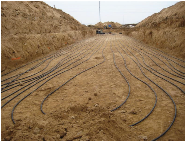
Figure 46. A typical racetrack horizontal loop geothermal field (left). This field served a 10,000 ft 2 fire station in Madison, WI. Figure 47. A typical slinky horizontal loop geothermal field (right). Photo credit: G.O. Loop, Randolph, WI.
