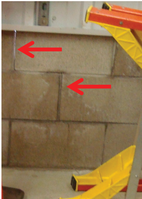
Figure 25. Cracks in the CMU blocking leading to high air infiltration.
