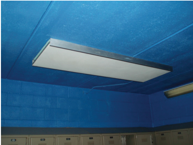
Figure 13. A radiant ceiling panel in the locker room (left).
