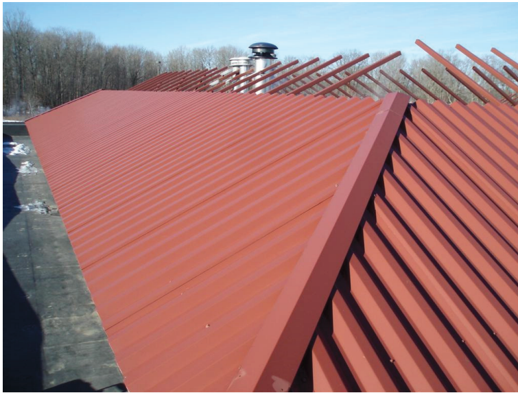
Figure 33. A photo looking at southwest-facing roof area #1 (camera looking north-northwest). This roof area experiences 2 percent average annual shading from some trees to the southwest. A pipe chase is located from the roof to the mechanical room where the vent pipes are sticking up over the architectural panels.
