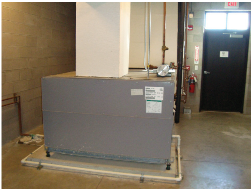
Figure 13. AHU-1 ventilation unit.
