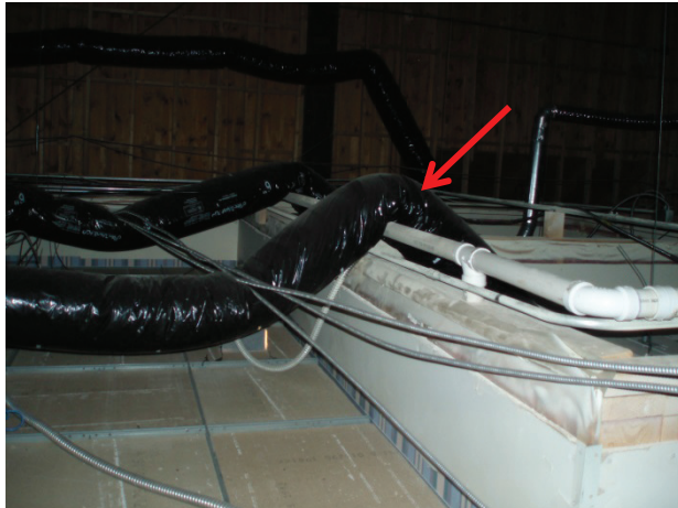
Figure 16. Typical flexible ductwork installed between the main supply trunk and the diffusers is not well supported and contains sharp bends.
