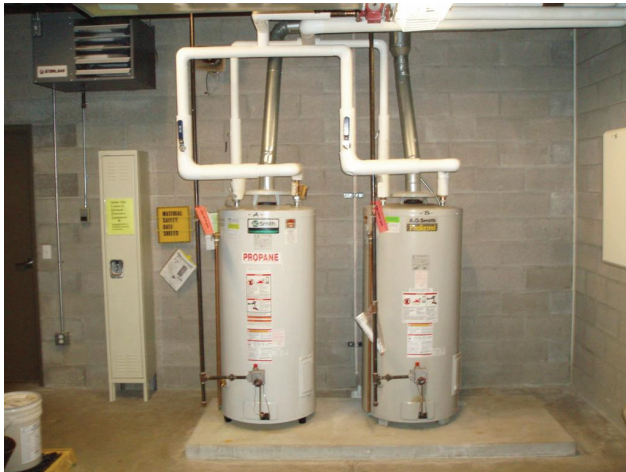
Figure 41. The propane water heaters in the mechanical room.
