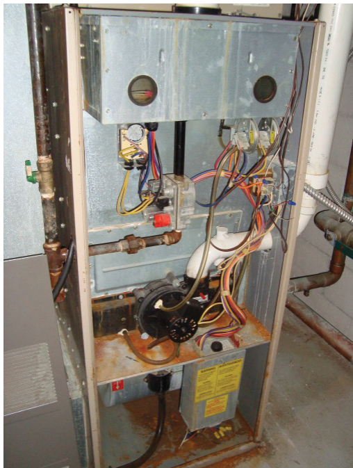
Figure 24. The weight room furnace shows a fair amount of rust and other moisture damage.
