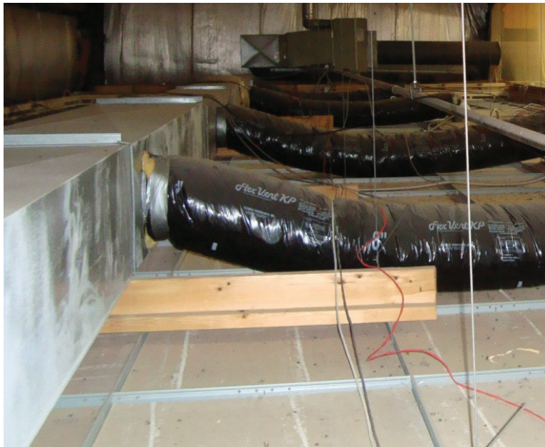
Figure 28: Weight Room ductwork is supported by the ceiling grid.
