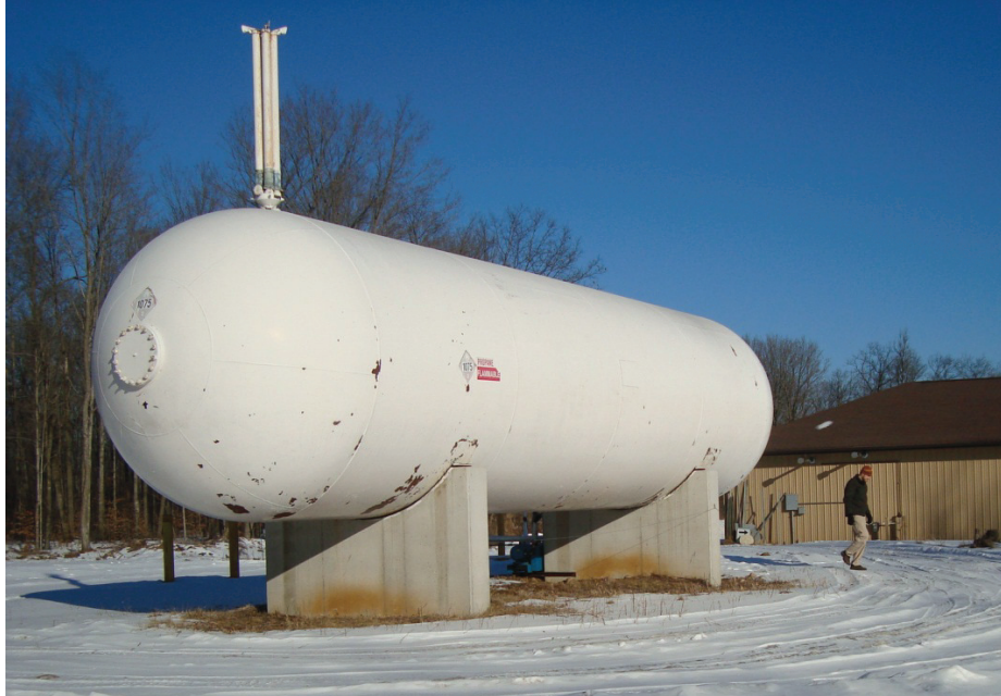
Figure 4. The 30,000 gallon propane tank.
