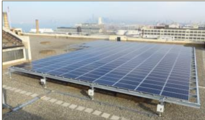
Figure A-65. 100 kW Solar PV Array at BAT
