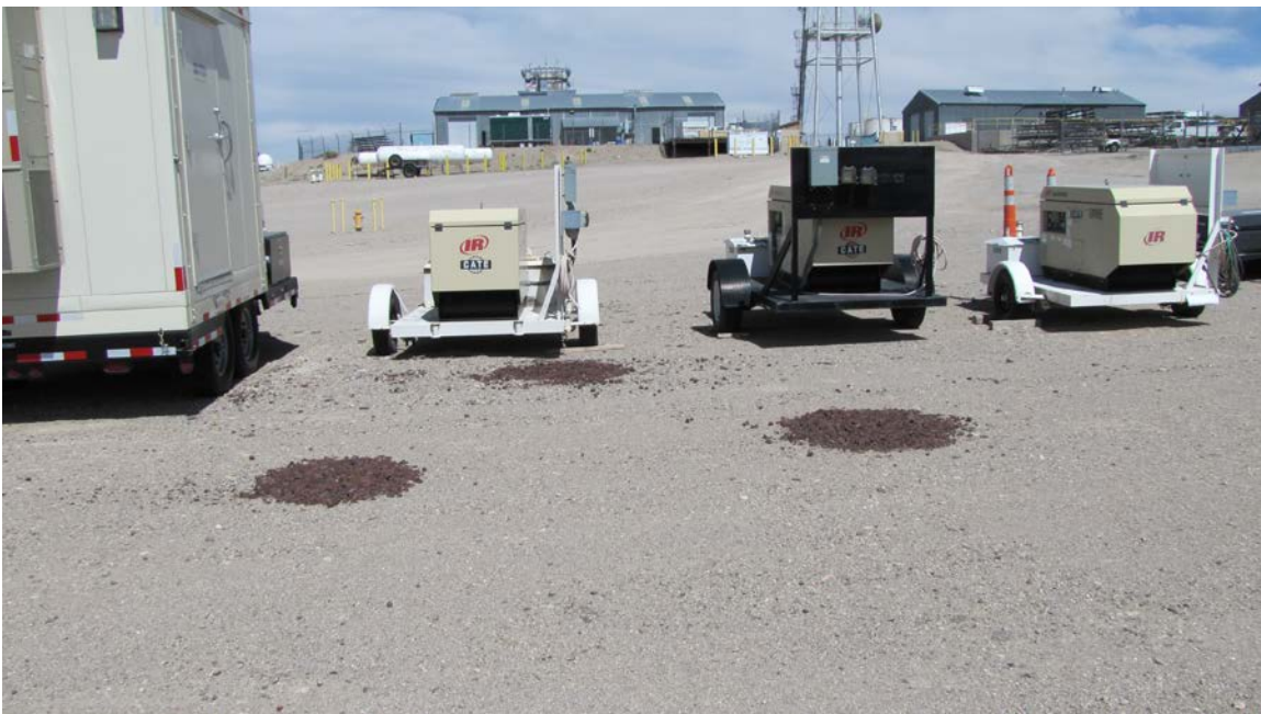
Photograph 6: CAU 424, Landfill Cell A3-3, Lava Rock Marking Surface Grade Monuments, 05/28/2014
