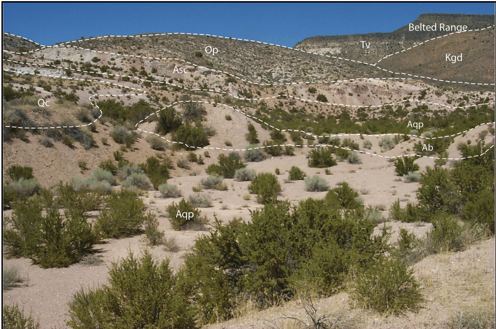
Figure 17. Quarry and borrow pit (Aqp) north of U15a area. Cut slopes (Asc) in Paleozoic bedrock (Op) and colluvium are visible. Prominent berm (Ab) has been pushed into place on borrow pit floor to control runoff.
