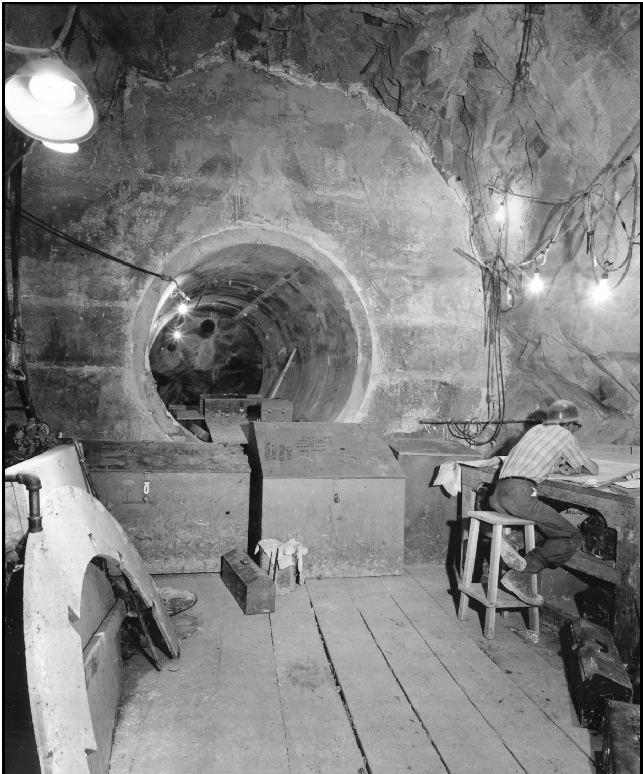
Figure 49. View of concrete experiment section and work station in the Pile Driver nuclear test (REECo photograph 3041-2, dated 1965, on file at the Nuclear Testing Archive, Las Vegas).
