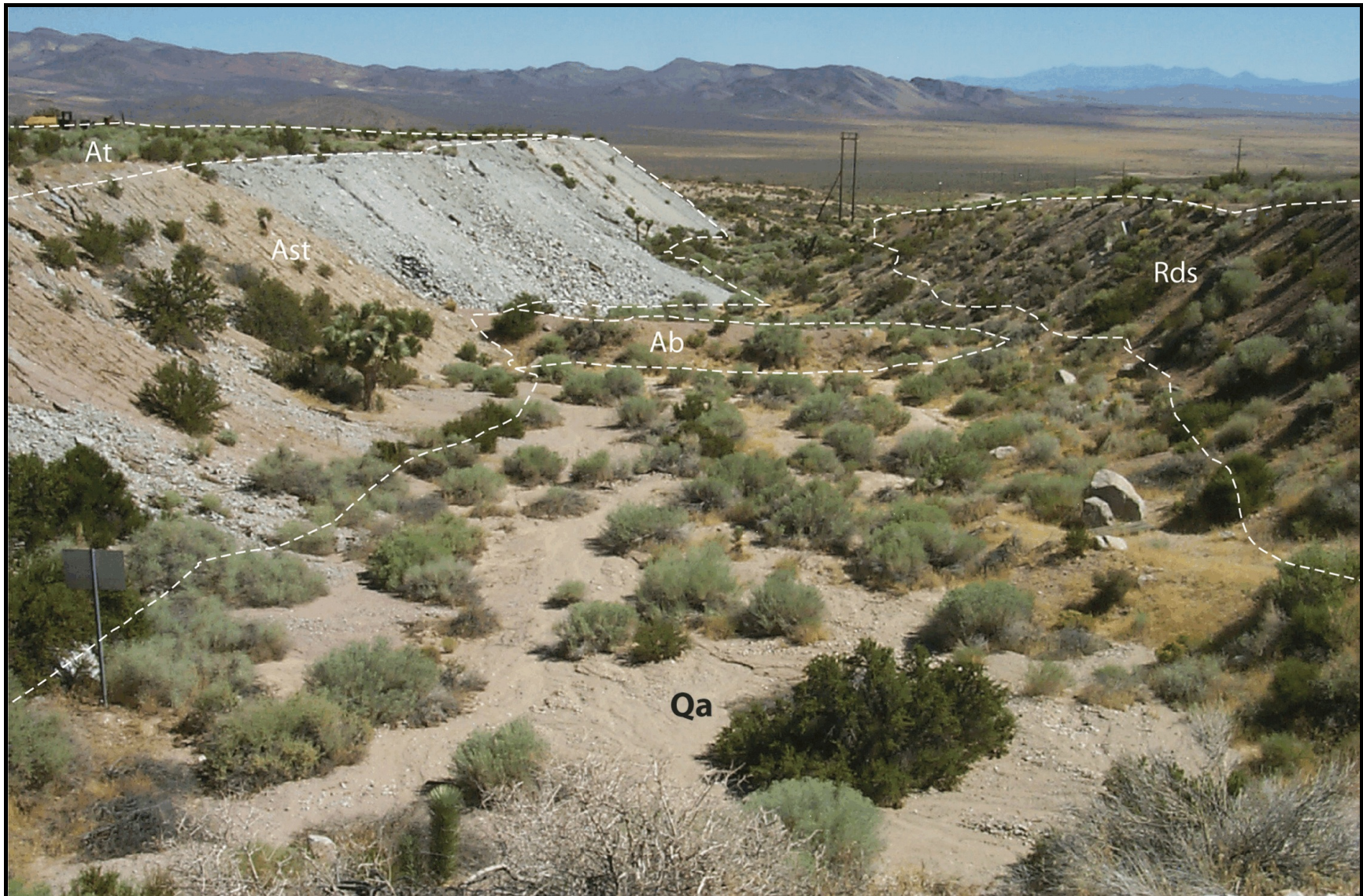
Figure 13. Alluvial valley partially filled with the muckpile (At and Ast) on the left and road side-cast (Rds) on the right. Also visible is active alluvium (Qa) and a prominent berm (Ab) placed across the stream to control runoff.
