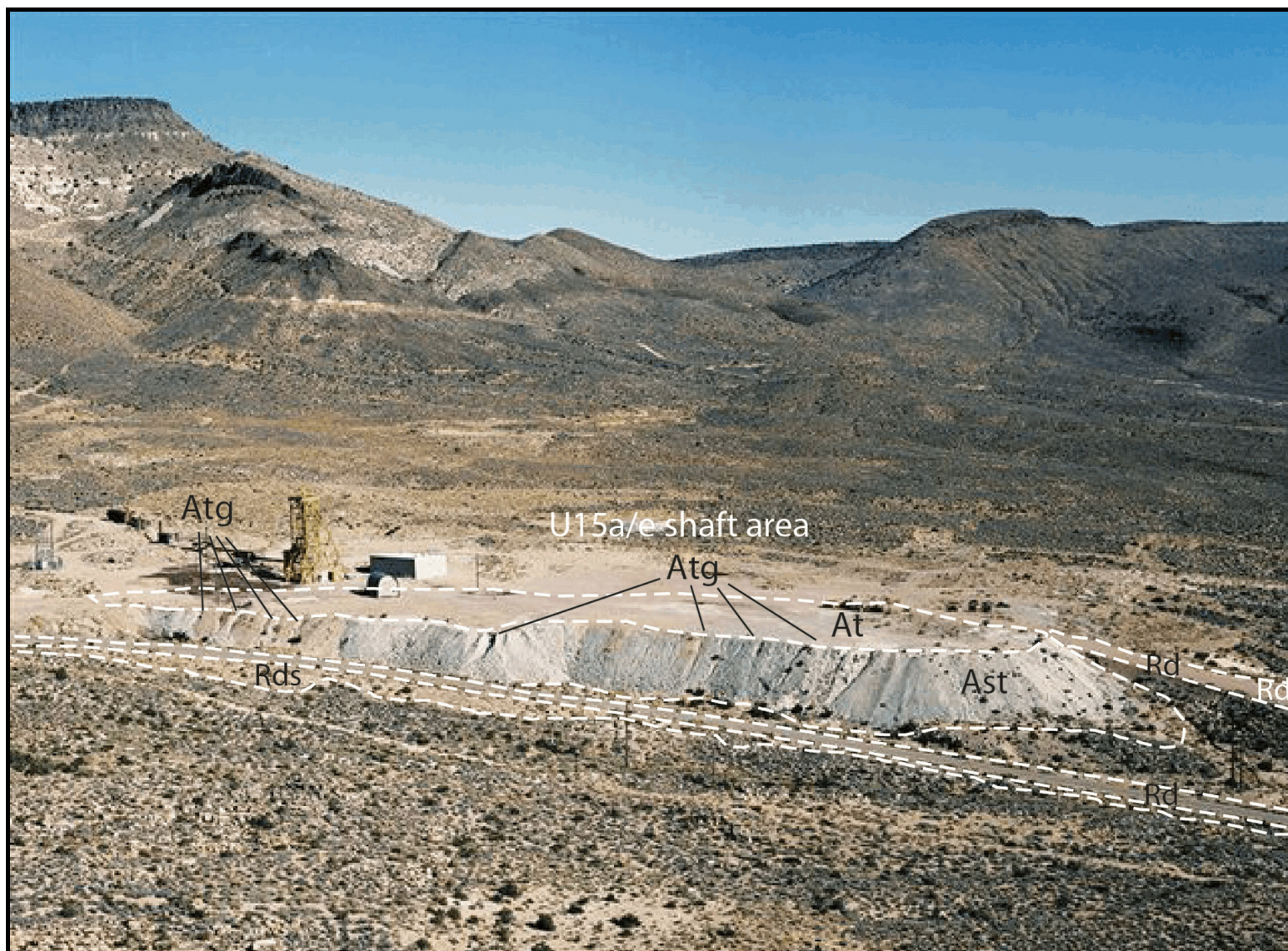
Figure 12. View northeast of the muckpile (At). Shown are rilled and gullied muckpile (Atg) on the muckpile slopes (Ast). Also visible are roads (Rd) and road side-cast (Rds).
