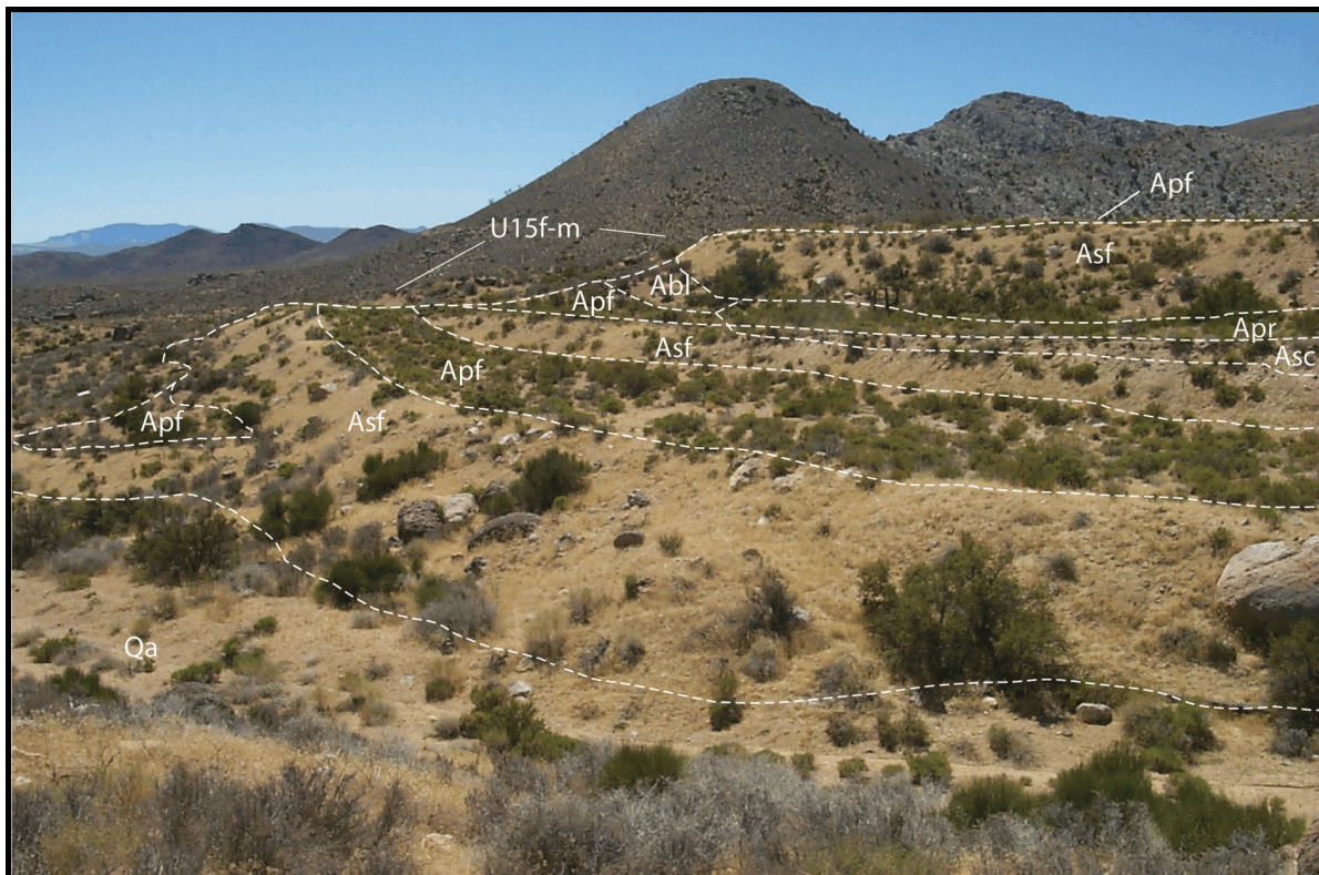
Figure 15. Constructed pad (Apf) and fill slopes (Asf) near the Pile Driver test (top); and fill pads and benches cut in fill (Apf) and pediment surface (Apr) in the U15f-m series area (bottom).
