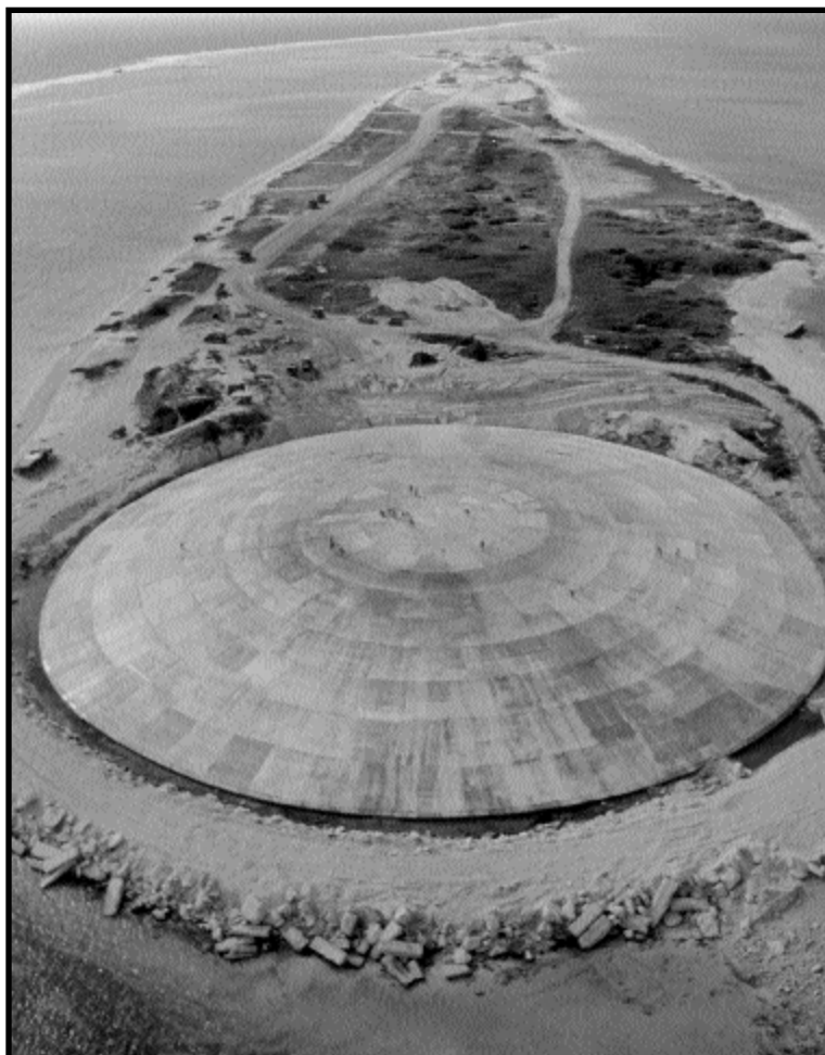
The Cactus Dome at Runit Island. Beneath this concrete dome on Runit Island (part of Enewetak Atoll), built between 1977 and 1980 at a cost of about $239 million, lie 111,000 cubic yards (84,927 cubic meters) of radioactive soil and debris from Bikini and Rongelap atolls. The dome covers the 30-foot (9 meter) deep, 350-foot (107 meter) wide crater created by the May 5, 1958 Cactus test. Note the people atop the dome. Enewetak Atoll, Marshall Islands. Photo circa 1990. Source: Defense Special Weapons Agency.
