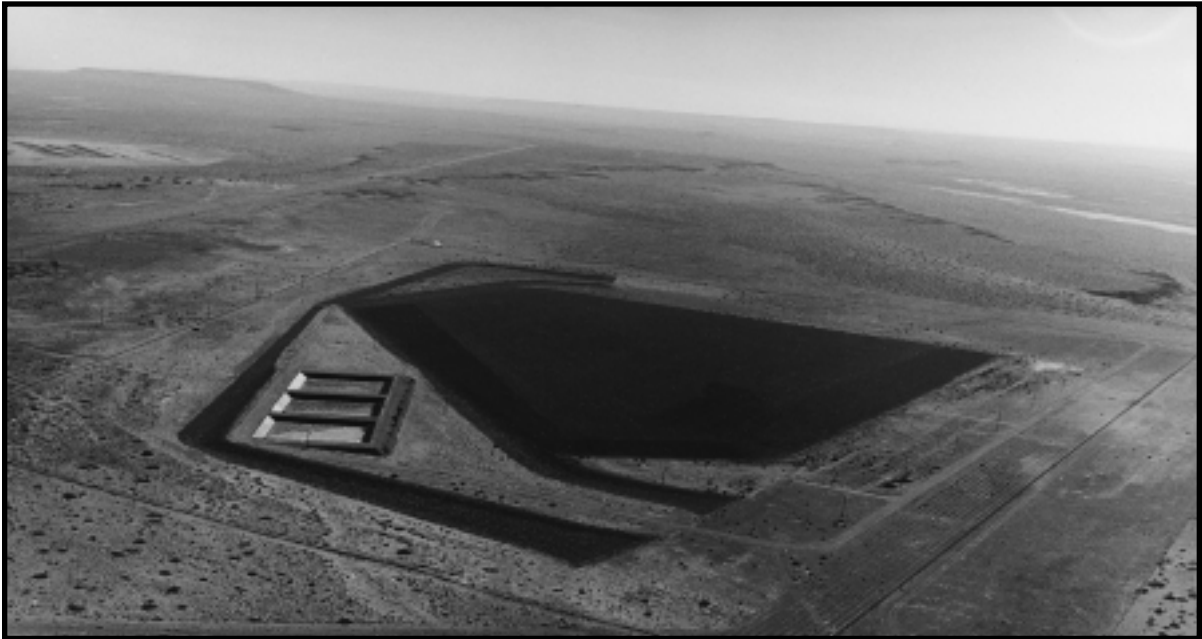
Tuba City Disposal Cell, Arizona. A total of 1,100,00 cubic meters of contaminated materials was stabilized onsite in a 50-acre disposal cell. The disposal cell has a radon barrier cover and rock surface layer to control erosion. Long-term surveillance and monitoring activities at the disposal cell include annual surface inspections and a 10-year revegetation program. The Tuba City Site consisted of 42 acres. Nine acres were covered by the uranium mill tailings pile, 18 acres were former evaporation ponds, and the remaining acres were contaminated by wind-blown materials. DOE will continue routine groundwater compliance monitoring after groundwater remediation is complete in 2010. Tuba City Uranium Mill Tailings Repository, Tuba City, Arizona, June 1998.
