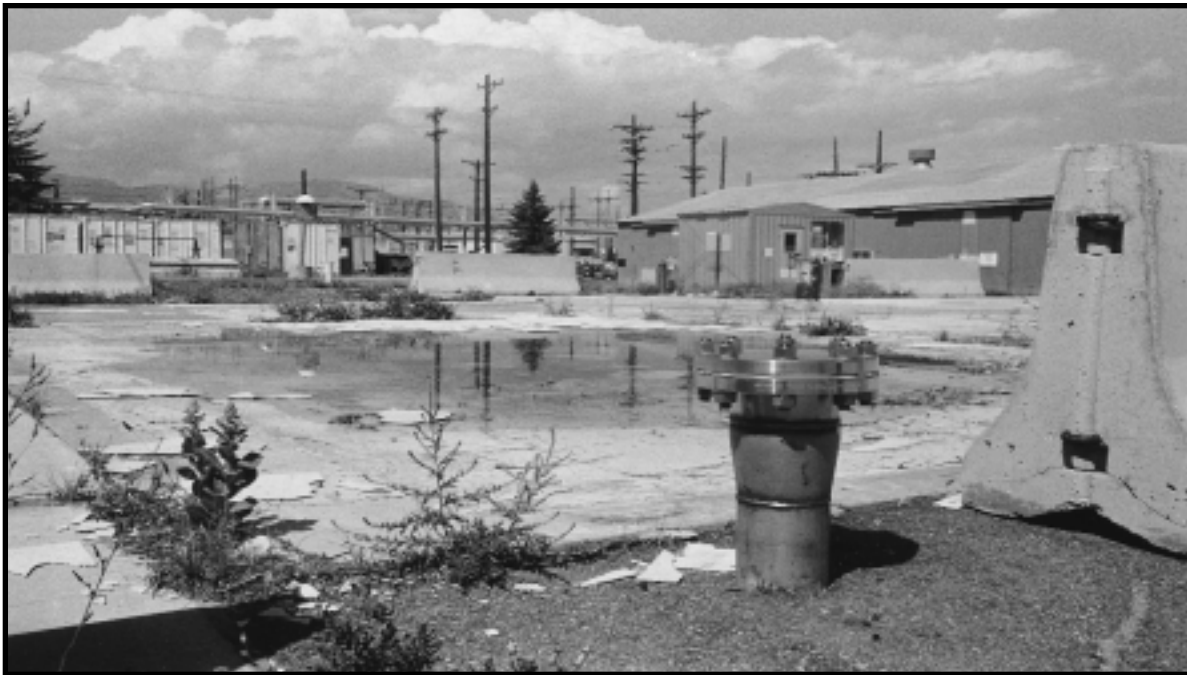
Remaining Foundation of Building 889 at the Rocky Flats Environmental Technology Site. The first radioactively contaminated building at the site to be demolished, this multi-purpose facility was a former uranium and beryllium waste repackaging plant that supported rolling and milling operations. Current plans call for virtually all of the facilities at Rocky Flats to be demolished and rubble to be disposed of appropriately. Foundations and utilities will remain in place unless removal is necessary to remediate underlying soil. Subsurface utilities between facilities will be capped and left in place. Future use options for this portion of the site include open space or light industrial uses. Rocky Flats Environmental Technology Site, Colorado, September 1999.
