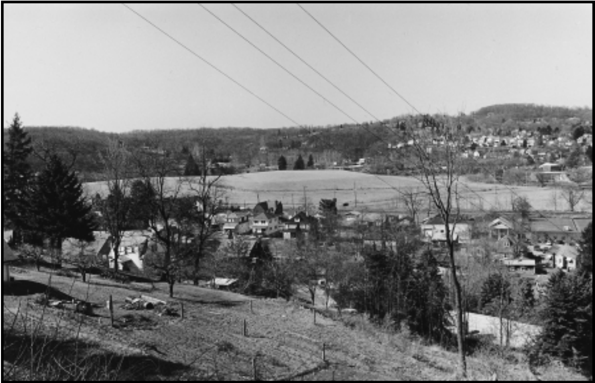
Canonsburg Disposal Cell. The 30-acre uranium mill tailings disposal cell in the center of the photograph is located in a residential area approximately 20 miles from Pittsburgh, Pennsylvania. Remedial actions were completed in 1985, and groundwater has been monitored since 1986. Annual groundwater monitoring will continue until 2004, and other long-term stewardship activities such as annual inspections and periodic vegetation control will be required indefinitely. Passive stewardship activities will include ensuring site access and groundwater use restrictions are maintained. Canonsburg Disposal Cell, Canonsburg, Pennsylvania, March 1999.
