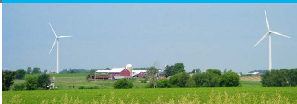
Photo by Ruth Baranowski, NREL/PIX 16410
