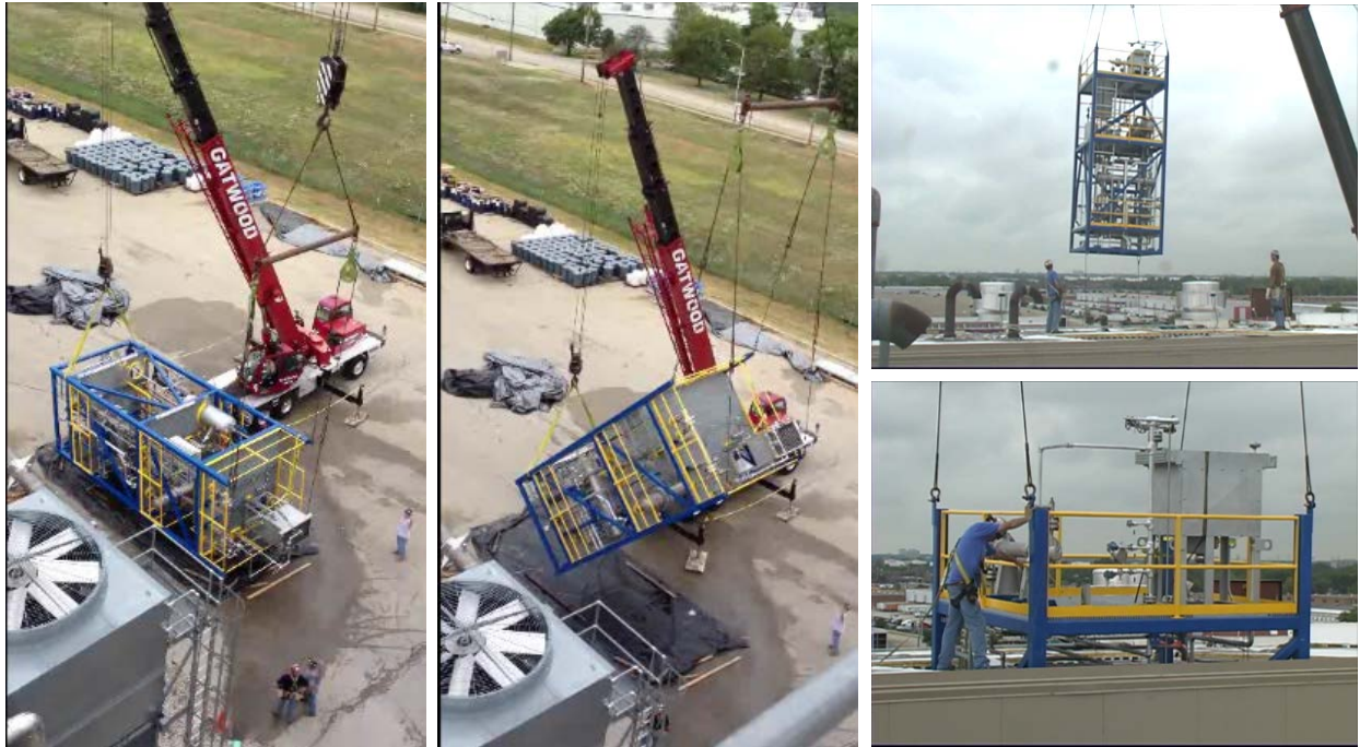
Figure 5-9 Lifting and Installing Top TIGAS Module, July 7, 2012
