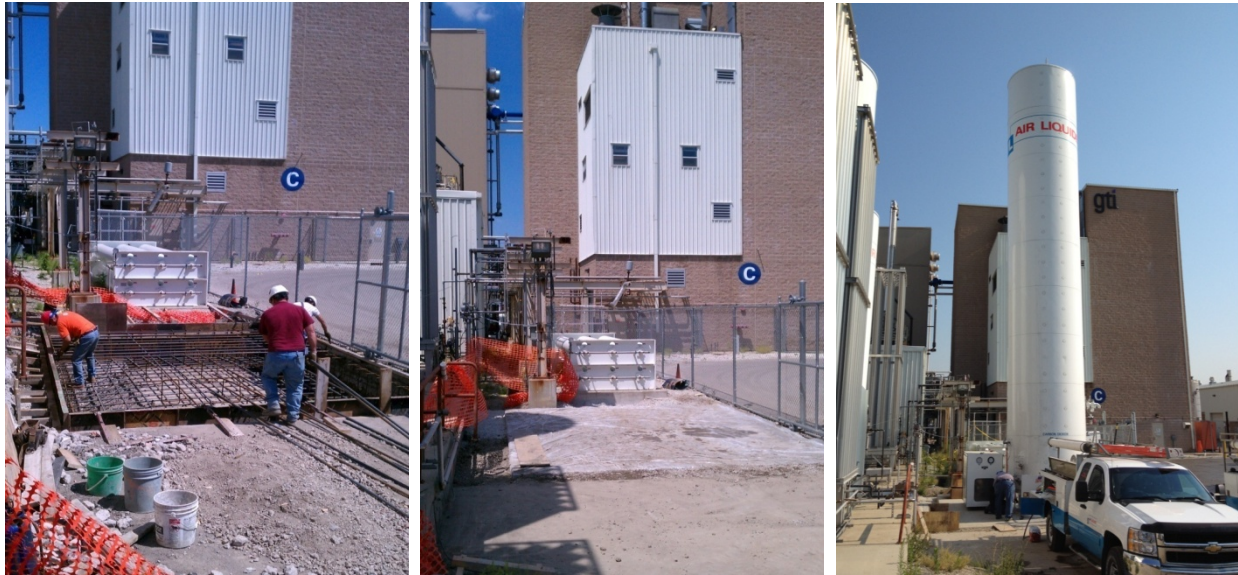
Figure 5-3 Carbon Dioxide Storage Tank Foundation and Installation, July 2012
