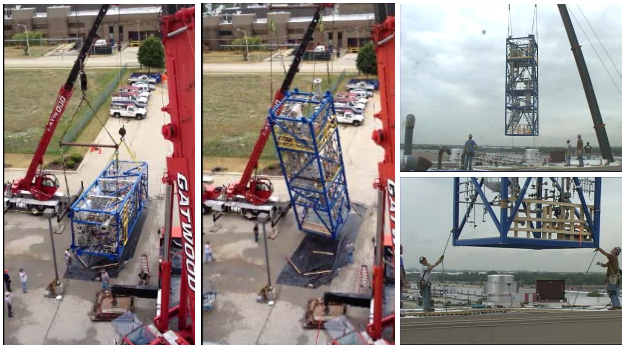
Figure 5-8 Lifting and Installing Bottom TIGAS Module, July 7, 2012
