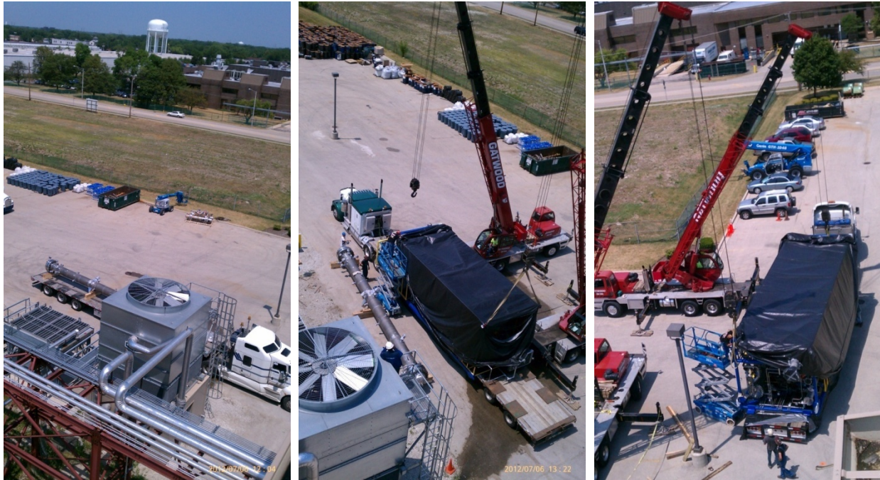
Figure 5-7 Delivery of TIGAS Modules (DME Reactor, Bottom Skid, Top Skid), July 6, 2012
