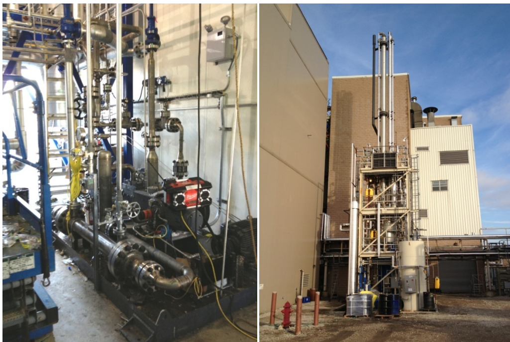
Figure 5-11 TIGAS Recycle Compressor & AGR with Upgrades, October 2012
