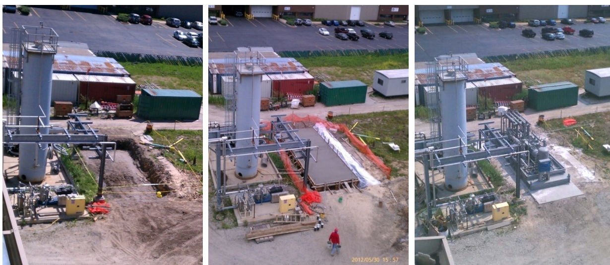
Figure 5-2 Syngas Compressor Foundation and Installation, May-June 2012
