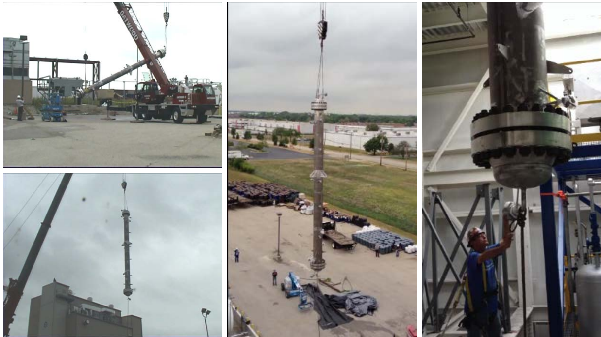
Figure 5-10 Lifting and Installing DME Reactor, July 7, 2012
