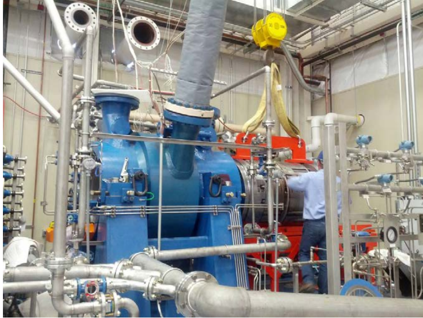
Figure 4-47. Photo of Bundle Removal to Repair Internal Seals
