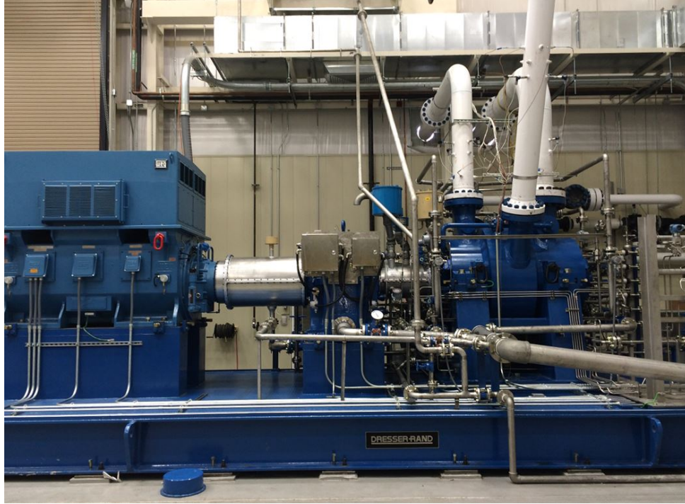
Figure 4-40. Installed Dresser-Rand Datum Compressor Package
