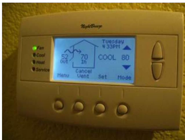
Image 41 - P9 NightBreeze Ventilative Cooling Controller
