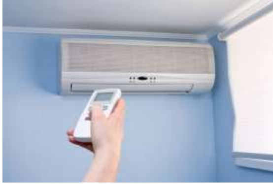
Figure 45 - Wall unit of mini-split heat pump. Source: www.drenergysavervirginia.com
