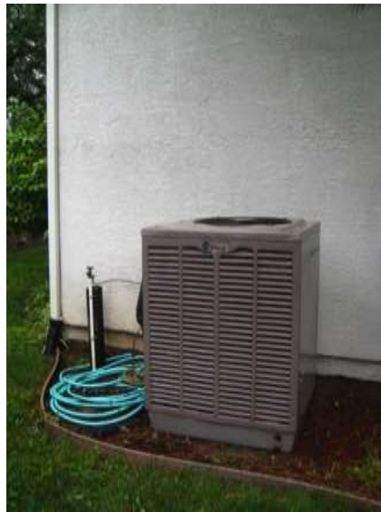
Image 40 - P9 Outdoor Evaporatively Cooled Condensor
