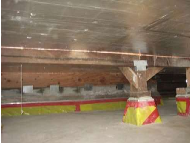
Image 30 - P7 Crawlpace with New Slab, Foam Board Insulation, Structural Reinforcement, Air Sealing and Water Proofing
