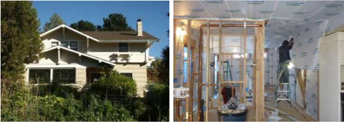
Image 28 - P7 Front of Home and House-Within-A-House Insulating
