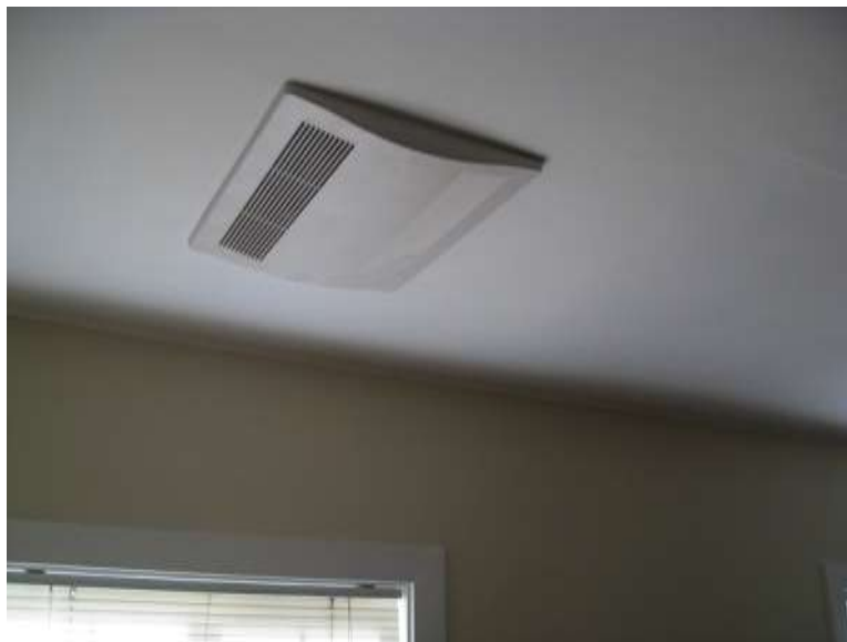
Image 48 - P5 Ceiling Mounted ERV
