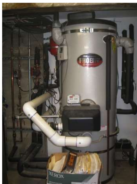
Image 44 - P10 Solar Combisystem Tank in Garage
