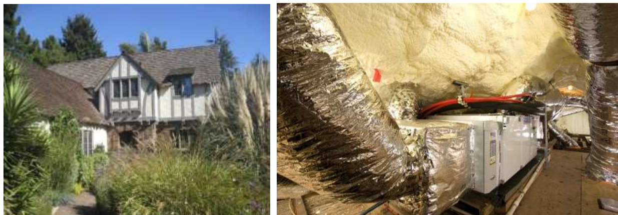
Image 3 - P2 Post-Retrofit Exterior and Insulated Attic
