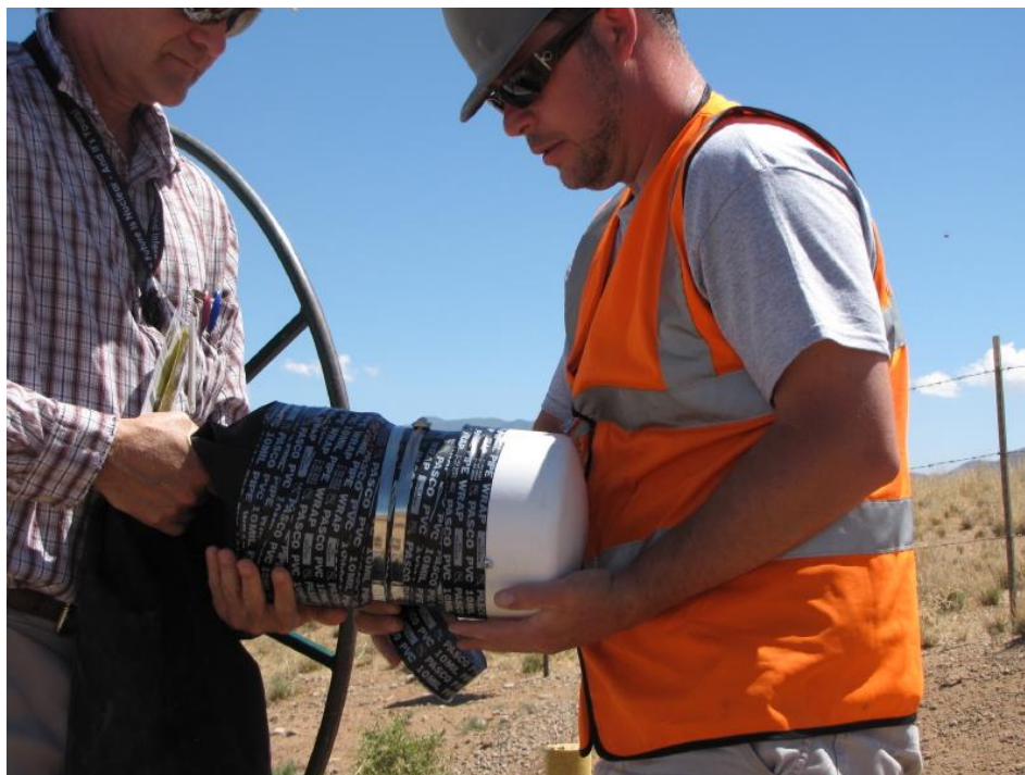
Figure F-5 Attaching the bottom weight to the lower end of the FLUTe™ borehole liner for soil-vapor monitoring well MWL-SV04.
