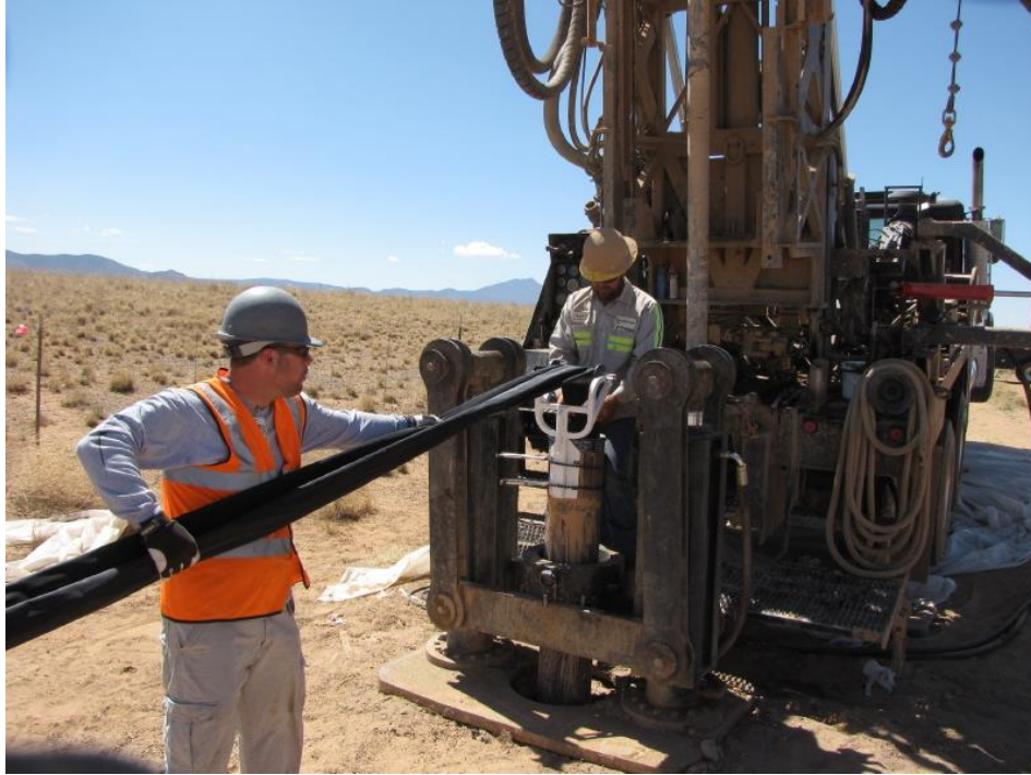
Figure F-3 Inserting FLUTe™ borehole liner into the drive casing for soil-vapor monitoring well MWL-SV03.
