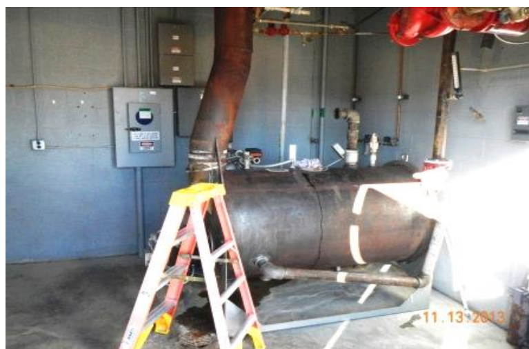
Building 03-57 Mission Control Center and Building 03-73 Boiler Room after asbestos abatement operations
