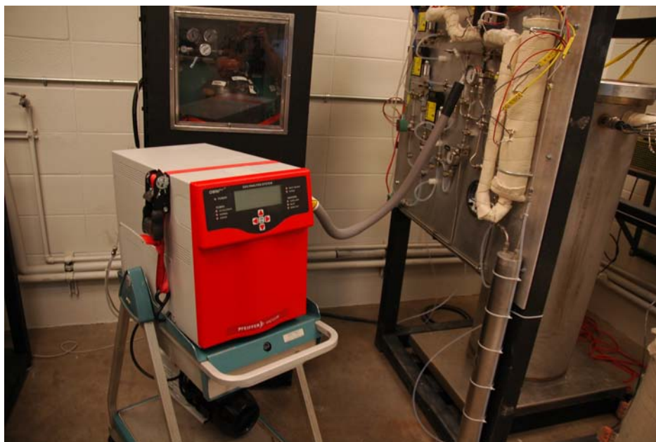
Figure 3.21: The GSD 320 tied into the effluent stream for the large batch purification.
