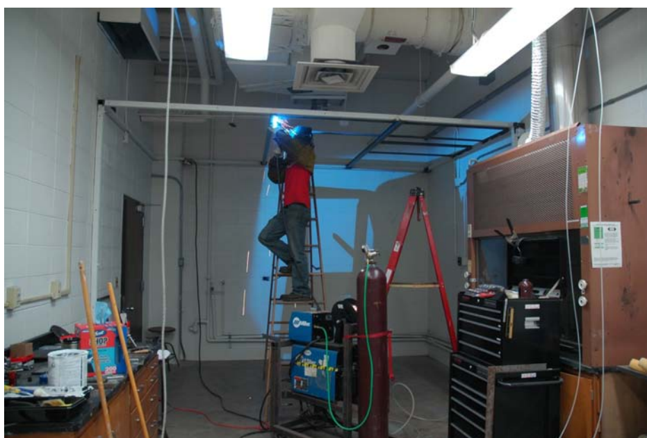
Figure 3.4: The room in the initial stages. Cross beams were MIG welded.
