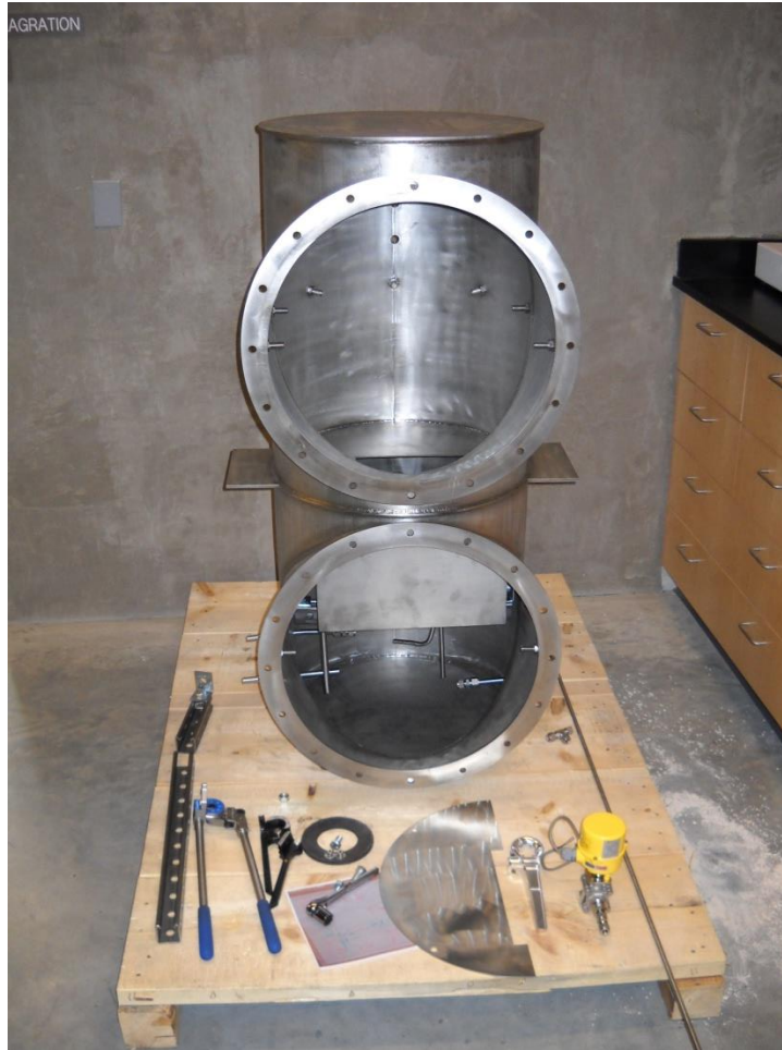
Picture 12. Fabricated Instrumentation Tank waiting for final positioning
