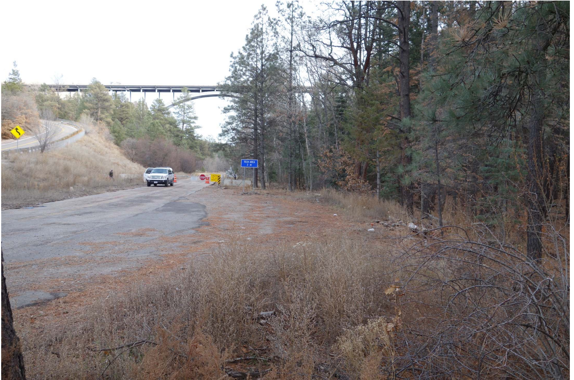
Photograph 2. Looking east at the area.
