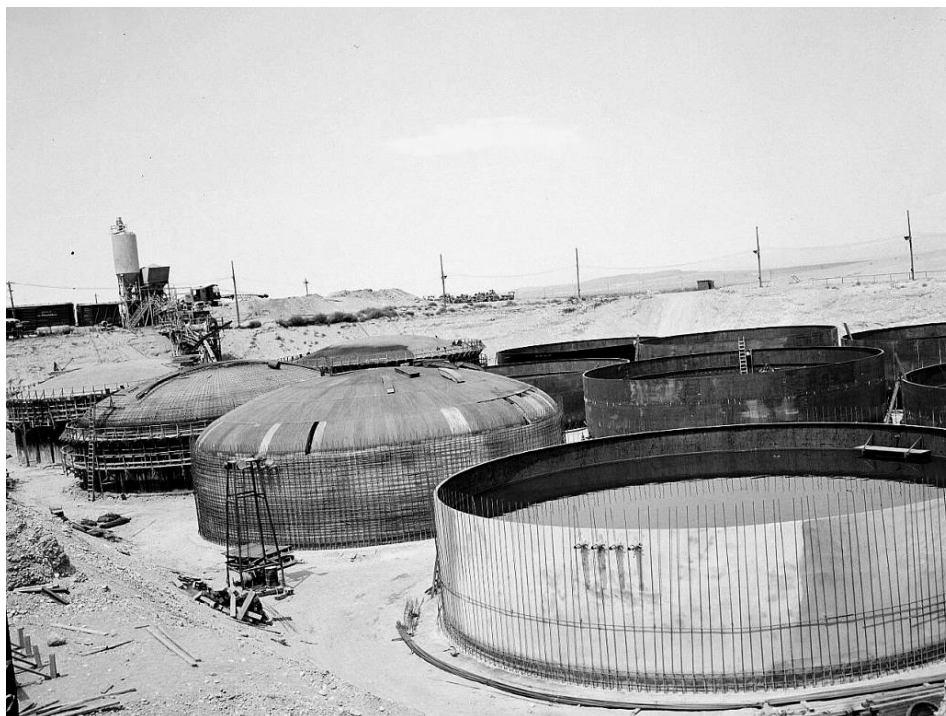
Fig. 1. 241-BX Tank Farm under Construction in 1947
