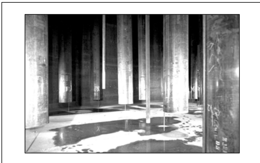
Fig. 5. Tank AY-102 Interior with Airlift Circulators
