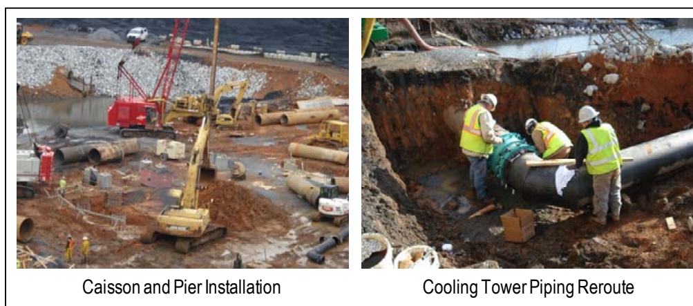
Figure 35. PC4 Site Preparation Work.
