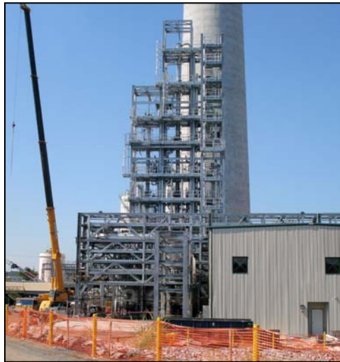
Figure 38. Installed PSTU Structure.
