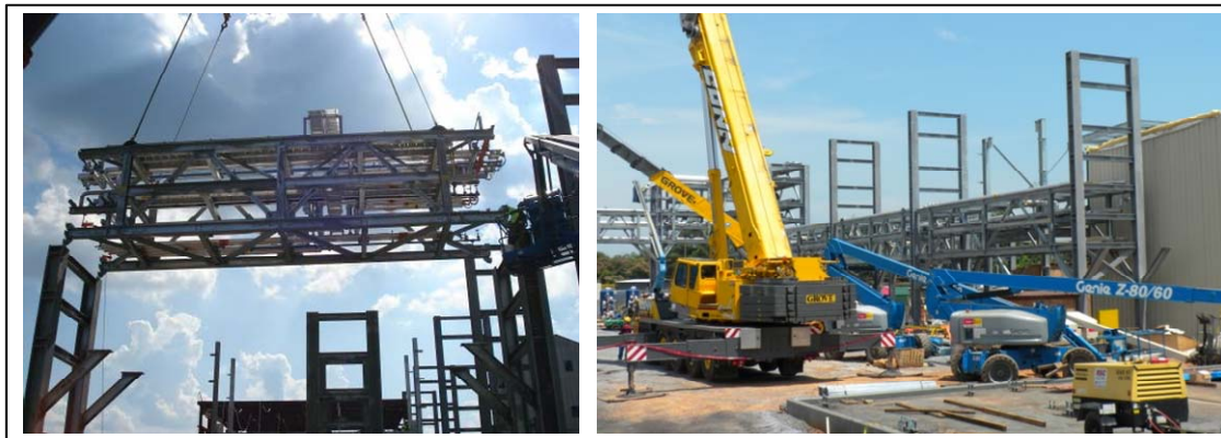
Figure 37. Installation of PC4 Utility Bridge.
