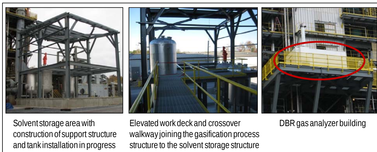
Figure 11. Construction of DBR Support Equipment.
