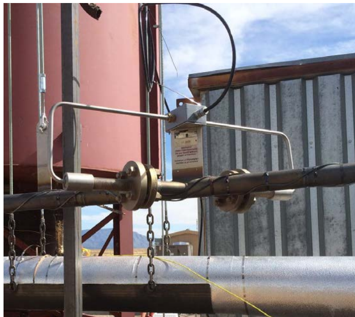
Figure 10: Flowmeter electronics are mounted separately, away from the heat.
