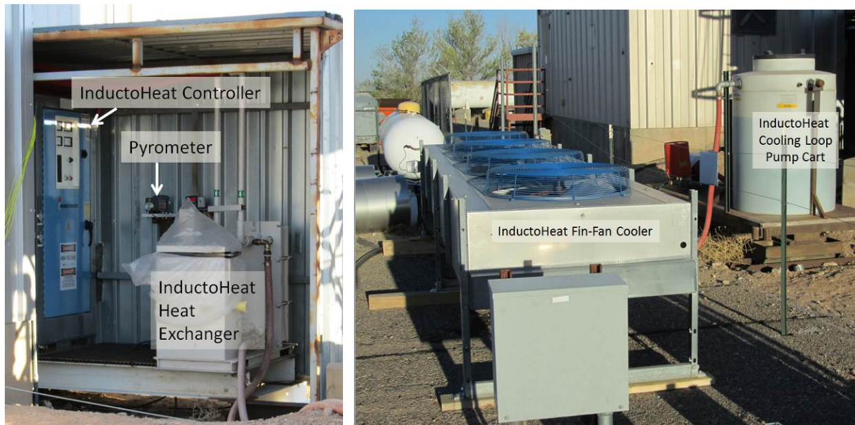
Figure 6 - The Electronics enclosure 1) contains the InductoHeat controller, pyrometer, and heat exchanger (left), and 2 is attached to the Cooling Loop and Cooler (right).
