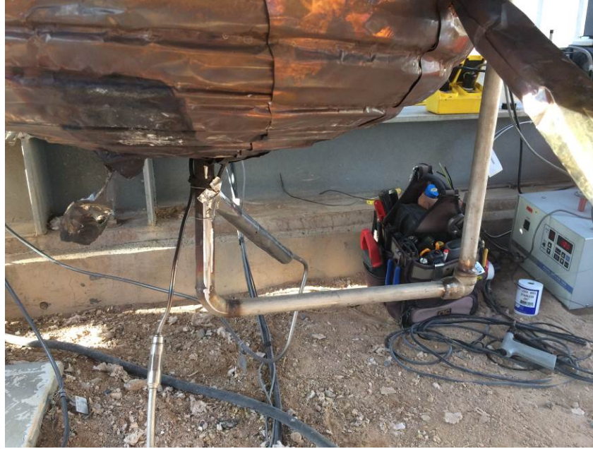
Figure 20: 3/4-inch drain line attached to bottom of tank to reintroduce salt to tank inventory
