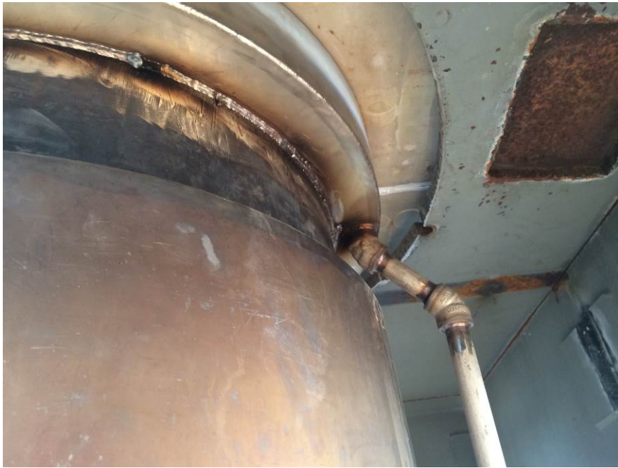
Figure 18: Catch pan attached to tank and 3/4-in drain line
