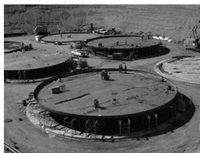
Secondary Liner Bottom
