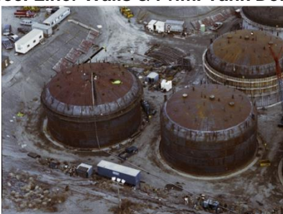
Primary Tank Hydrostatic Test
