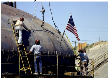
Secondary Liner Top Knuckle
