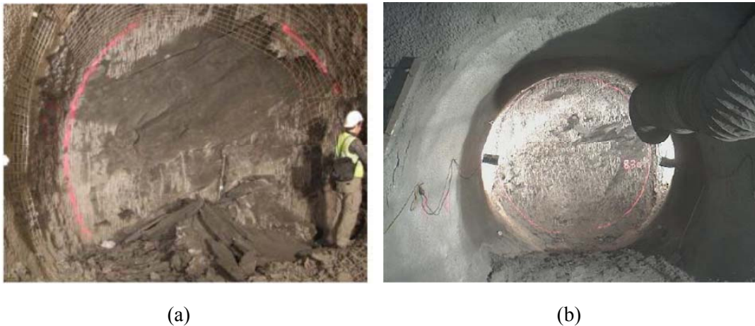
Figure 2-4. MB Niche 2 in construction: (a) the excavation advancing face, and (b) the view of the niche after reinforcement with shotcrete.
