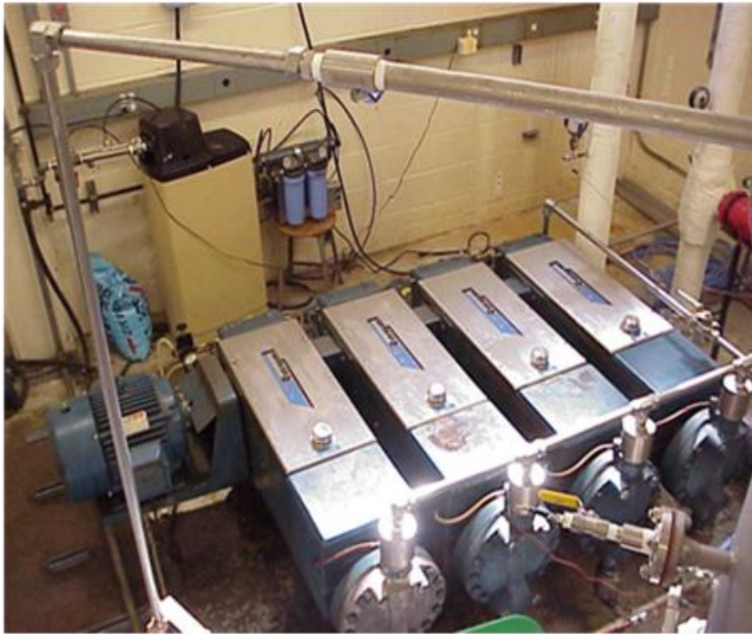
TOP LEFT AERIAL VIEW OF WATER PUMPS, PH CONTROL SYSTEM, PRESSURE RELIEF VALVE, FINE FILTER FLOW CONTROL VALVE, CHILLED WATER RETURN, AND CHILLED WATER SUPPLY
