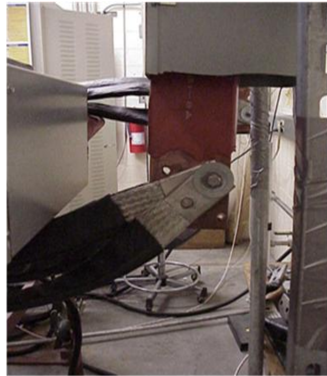
FLEXIBLE POWER CONNECTION TO POWER SUPPLY SOLID BUS BARS
