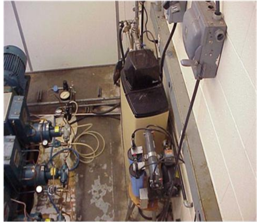
TOP AERIAL VIEW OF WATER PUMPS AND PRESSURE RELIEF VALVE, FLOW CONTROL VALVE AND PH CONTROL SYSTEM
