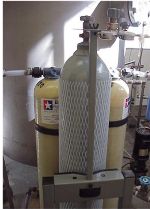
RIGHT SIDE VIEW OF NITROGEN TANK AND DEIONIZATION BEDS
