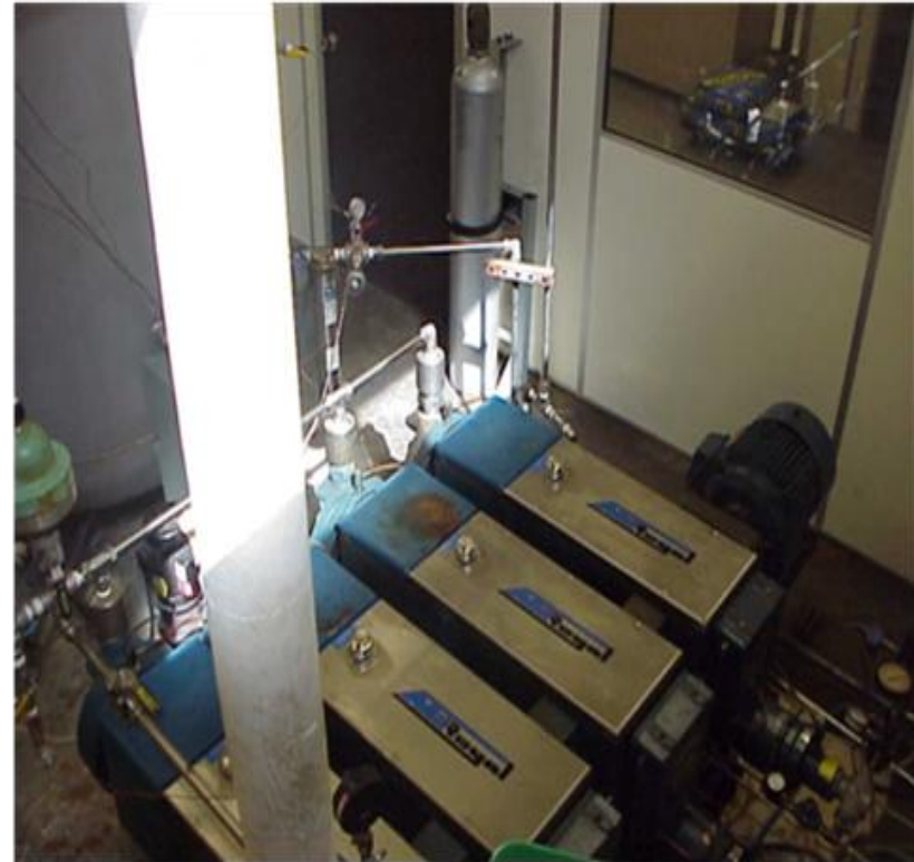
TOP AERIAL LEFT VIEW OF WATER QUALITY METER, WATER PUMPS & CONNECTIONS, PTC, PRESSURE STABILIZER, CHILLED WATER RETURN, PH CONTROL SYSTEM, FLOW CONTROL VALVE, & PUMP MOTOR
