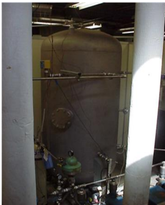
AERIALSIDE OF DEIONIZED WATER RESERVOIR, WATER QUALITYMETER, DEIONIZED BED FLOW LOOP, THERMOCOUPLES, PRESSURE STABILIZER, PTC
