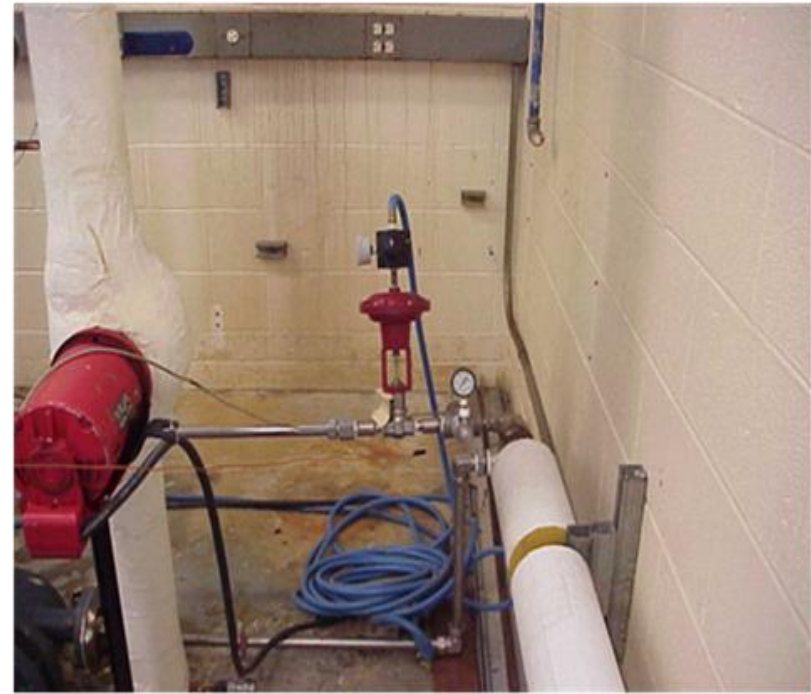
FRONT VIEW OF HEAT EXCHANGER, PUMP CONTROL, CONTROL VALVE, AIR PACK FILTER REGULATOR, COOLING WATER IN AND OUT TO DRAINAGE AND CHILLED WATER SUPPLY
