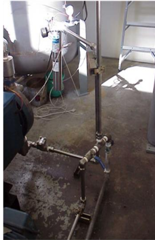
TOP FRONT VIEW OF FINE FILTER AND BYPASS VALVE
