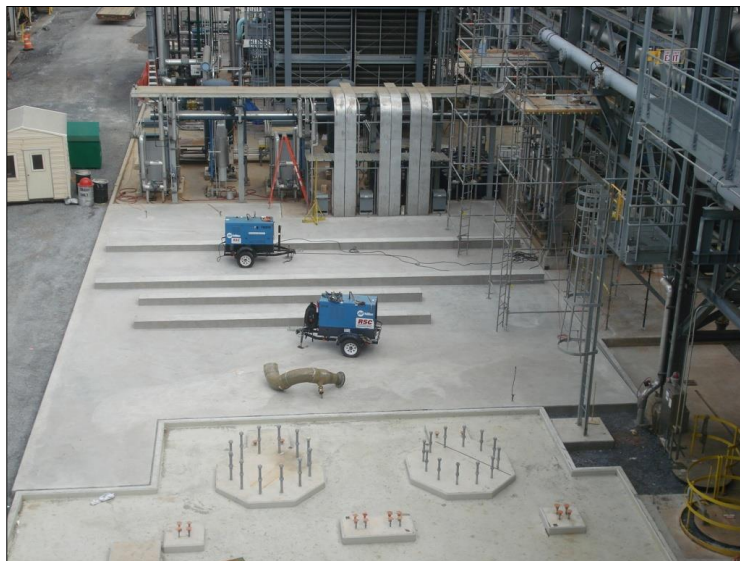
Figure 16. Pilot Bay 3 Foundation to Support MTR 20-TPD Unit
