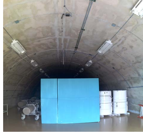
Figure 3 Interior view of Bunker 8013 showing north (left) and south sections
