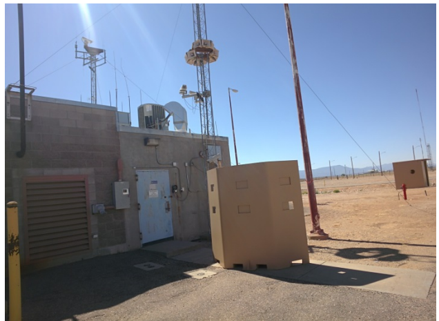
Figure 15 Communications and security features visible during walk-through
