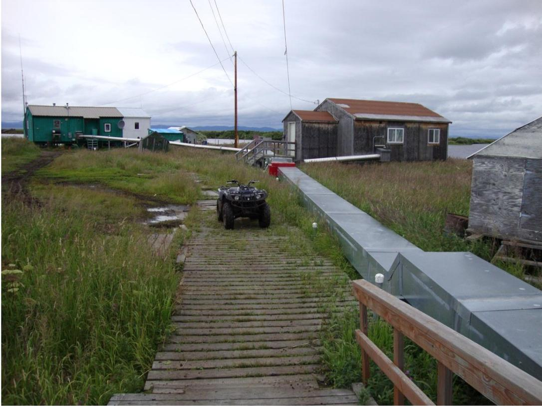
Photo 8: *Vacuum utilidor* with service line and arctic box in the background
