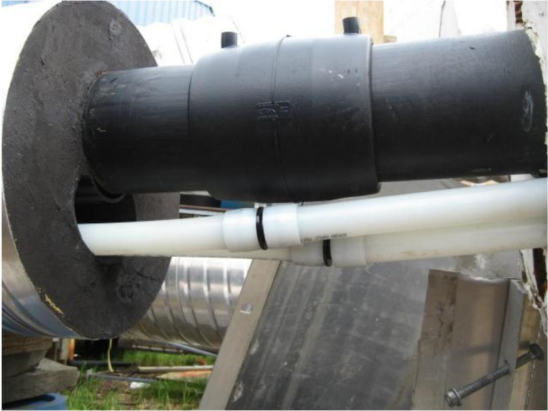
Photo 2: *New glycol heat trace piping installed*
