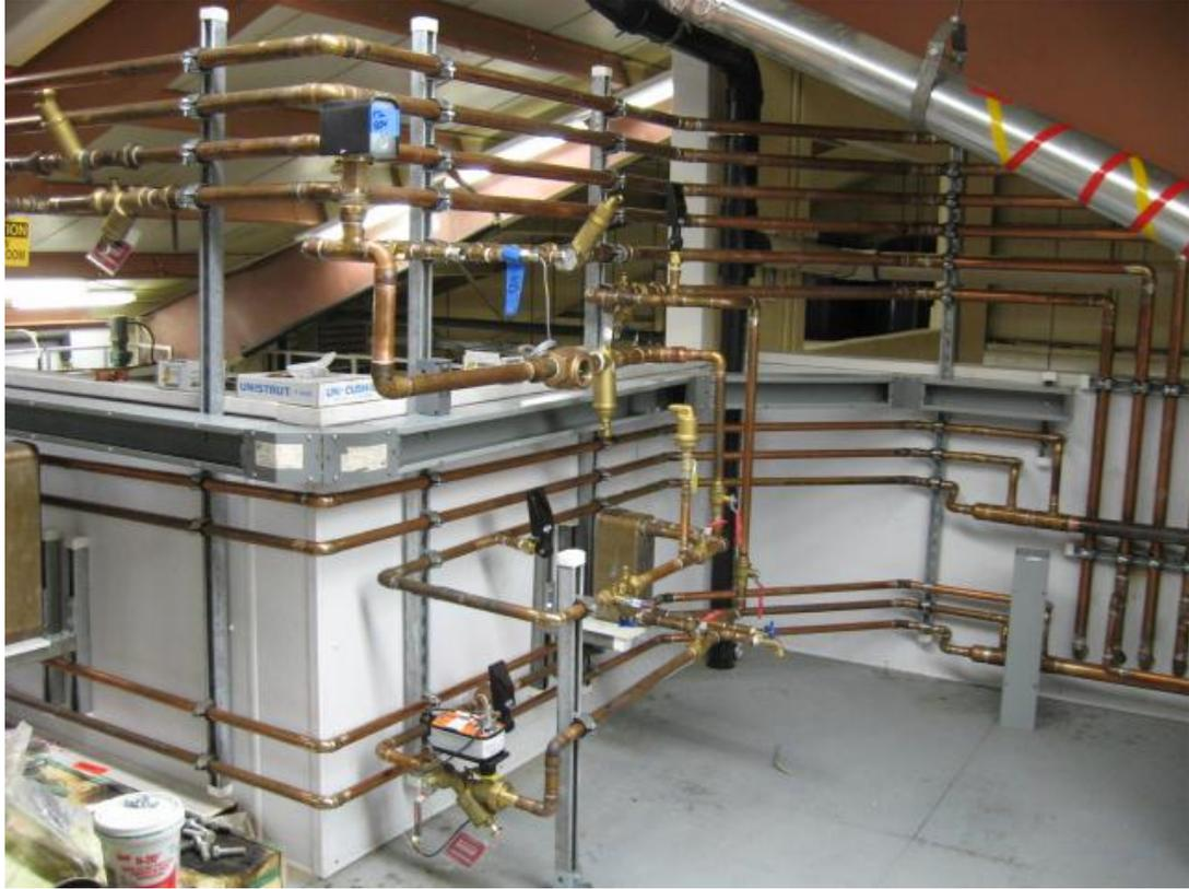
Photo 4: *Hydronic heat add piping in the water treatment plant before insulation was installed*
