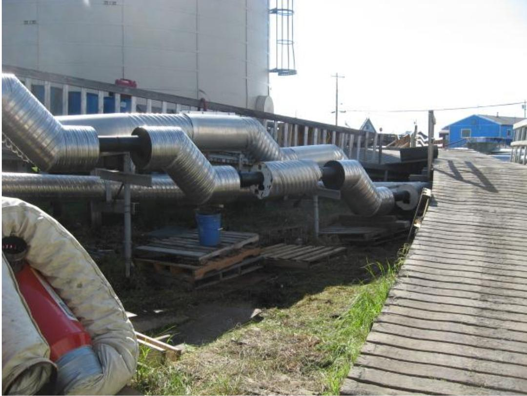
Photo 3: *Vacuum sewer main (realignment and heat trace installation underway)*
