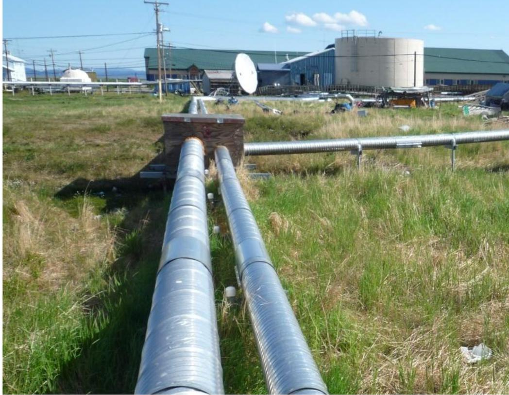
*Photo 7: Junction box – re-insulation of these boxes improved efficiency*
