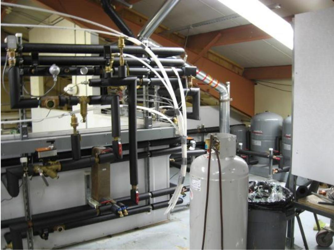
*Photo 5: Hydronic heat add piping in the water treatment plant after insulation was installed*
