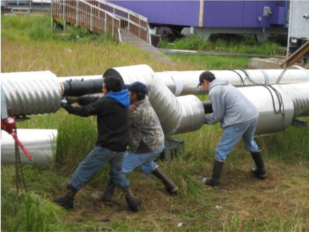
Photo 1: *Selawik crew pulling new glycol lines on the vacuum sewer main*
