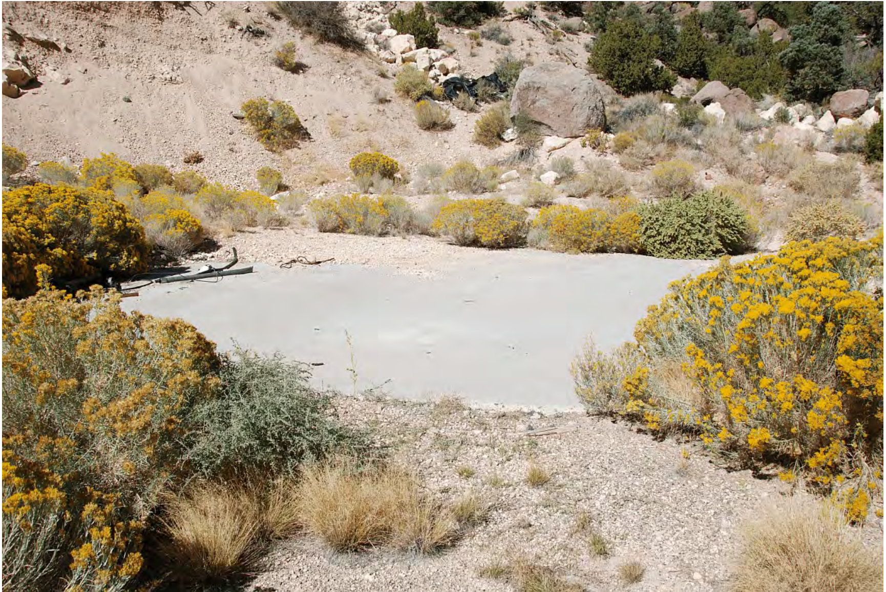
Figure 206. Feature 56, concrete foundation for the two air compressors, U12n Tunnel, view west (2008).
