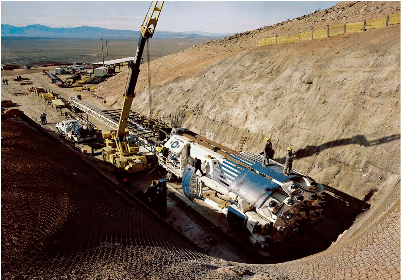
Figure 39. Tunnel boring machine at start of X tunnel in Area 25, 1982 (photograph MX-027-7, on file at Remote Sensing Laboratory).
