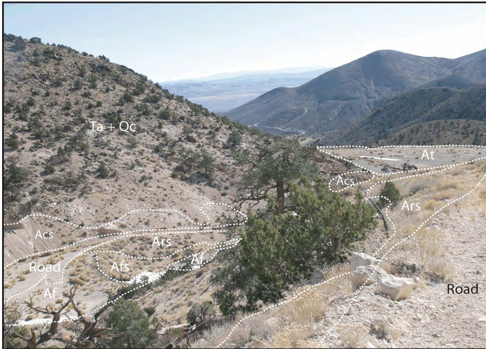
Figure 116. View east from the access road above the U12n Tunnel portal area showing the tailings (At), bedrock cut slopes (Acs), fill pads (Af) and fill slopes (Afs), and road side cast material.
