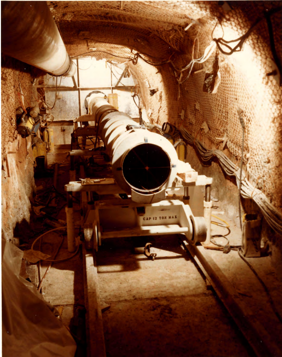
Figure 7. Installation of a line-of-site pipe section near the working point for the Huron Landing nuclear test, 1981 (photograph CAA-027-4, copy on file at NNSA/NSO Curation Facility, Las Vegas, Nevada).
