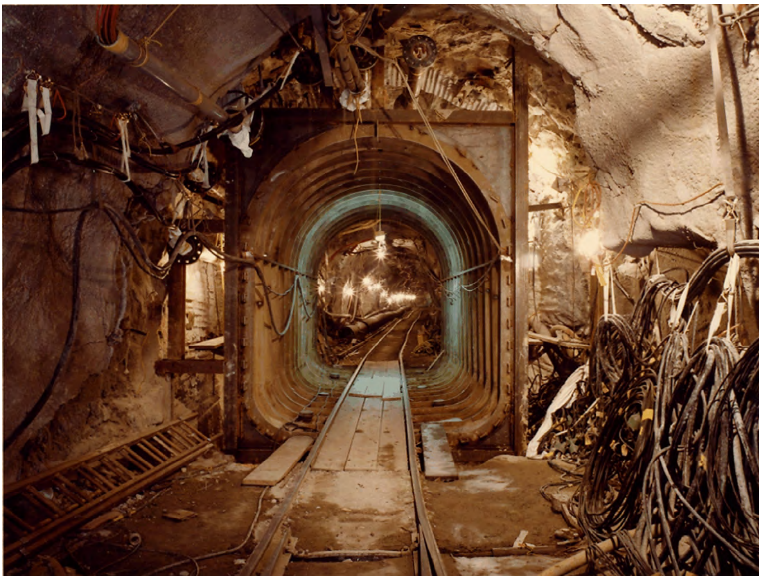
Figure 18. View toward portal of the trainway and overburden plug being constructed in the U12n.08 drift, 1982 (photograph CAA-092-14, copy on file at NNSA/NSO Curation Facility, Las Vegas, Nevada).
