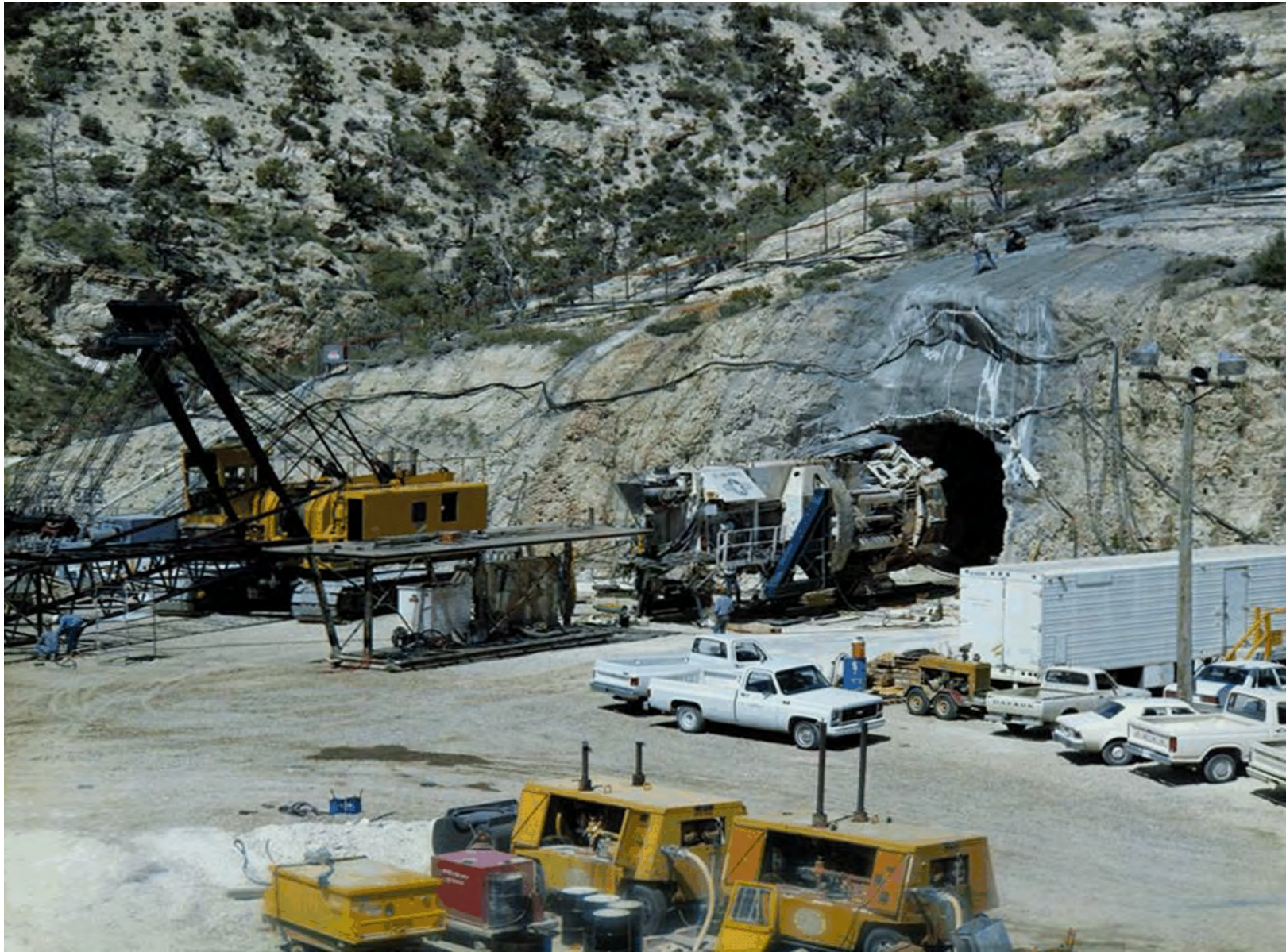
Figure 40. Tunnel boring machine at start of the extension drift for the U12n Tunnel (photograph courtesy of Wayne Griffin).
