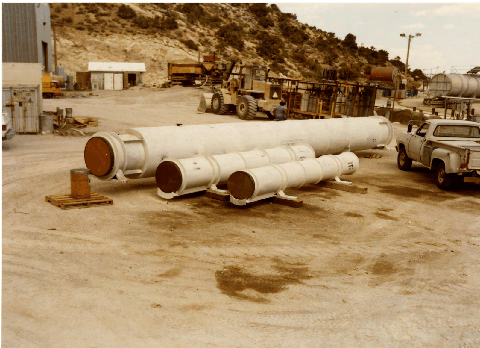
Figure 14. Line-of-sight pipe and muffler sections for the Huron Landing nuclear test, 1981 (photograph CAA-019-5, copy on file at NNSA/NSO Curation Facility, Las Vegas Nevada).
