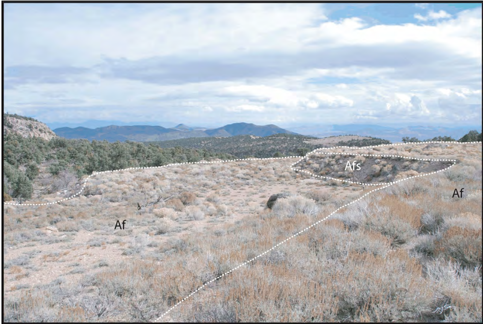
Figure 109. View of U12n.03 cable hole #1 on Rainier Mesa. Shown are broad area of terraced artificial fill (Af) and fill slopes (Afs).
