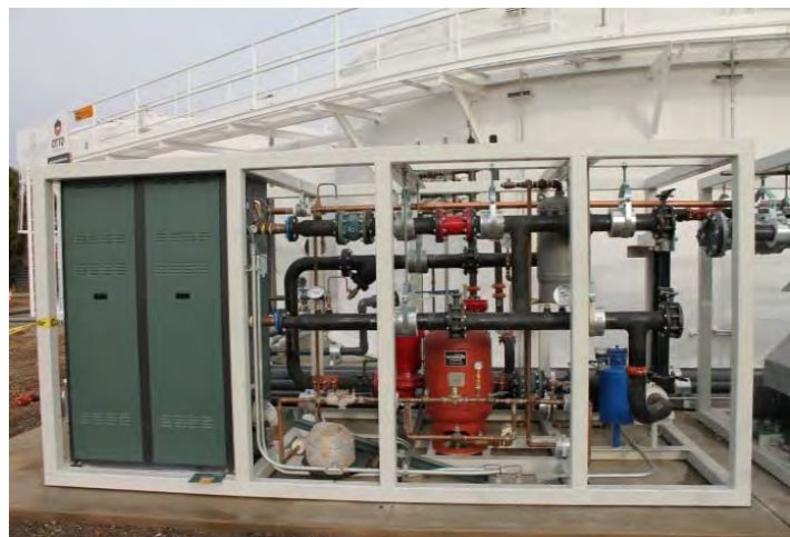
Figure 4 - CleanWorld's modular, prefabricated skids lower cost substantially.
