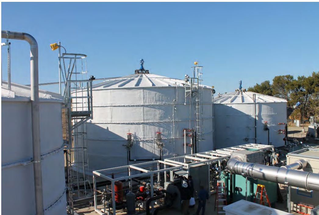
Figure 9 - Insulation Applied to Tanks
