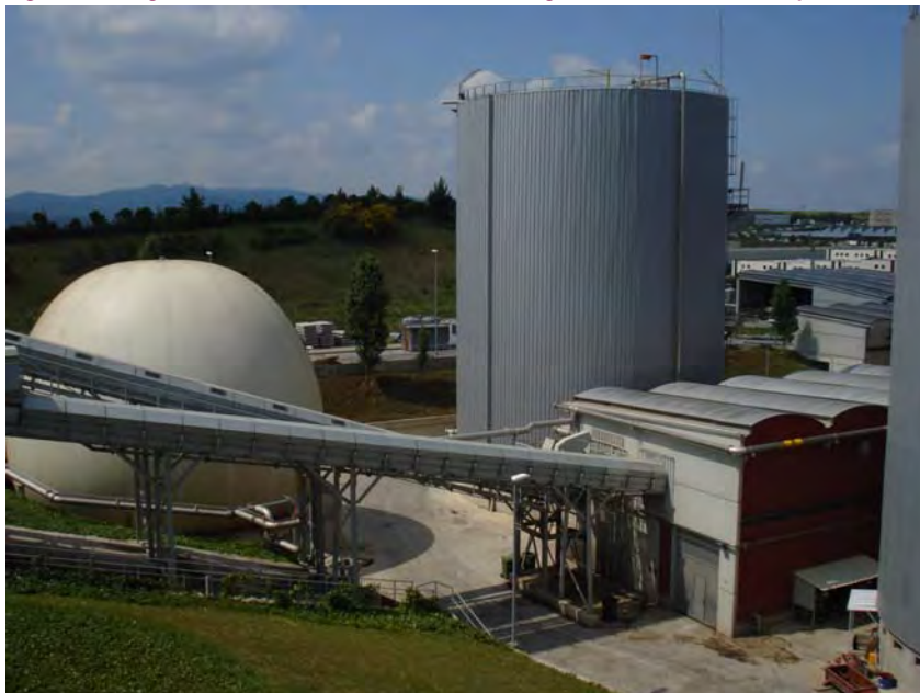
Figure 3. High-Solids Anaerobic In-Vessel Digestion, Barcelona Spain
