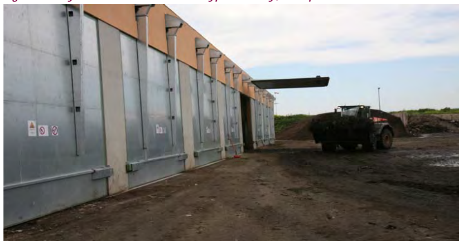
Figure 5. Dry Fermentation Bunker-Type Facility, Europe
