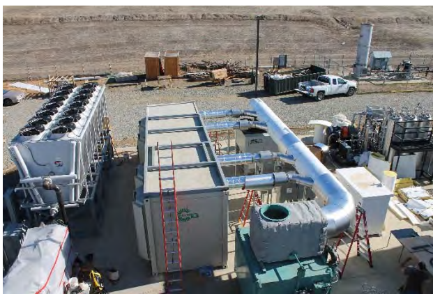
Figure 5 - Skid Mounted Gas Refining Equipment and Microturbine package at the READ Facility
