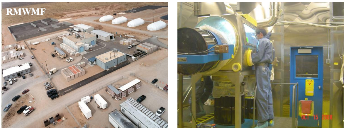
Figure 2.6 Aerial photograph (left) and glove box operations (right) at the RMWMF.
