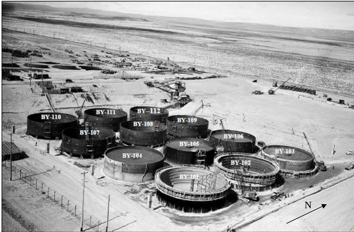
Figure 3-4 BY Farm Construction Photograph (N1D0000725)
