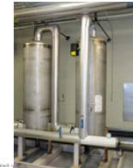
Static Filter (siloxane)
