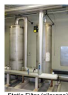
Static Filter (siloxane)
