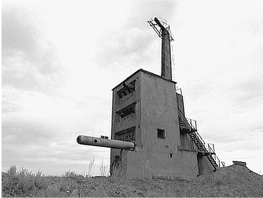
Figure 6. Instrumentation facility (“goose”) for physical observations with measuring equipment installed on top (in “cigar”).
