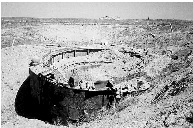
Figure 40. Remains of a missile launch silo destroyed by a conventional explosive charge.
