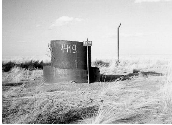
Figure 62. Exterior view of a shaft ready for an underground nuclear test.
