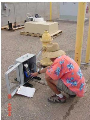
Sensors on-line collecting data at discrete locations within a water distribution system
