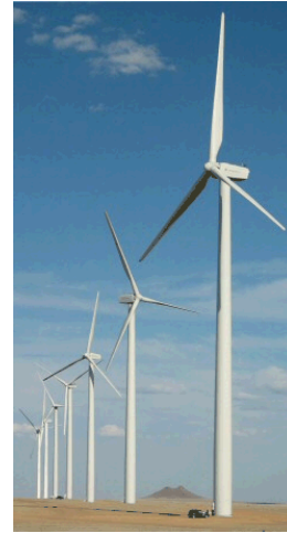
Figure 1. GE 1.5 MW Wind Turbines in the Colorado Green wind farm near Lamar, Colorado. The item at the base of the closest turbine is a minivan.
