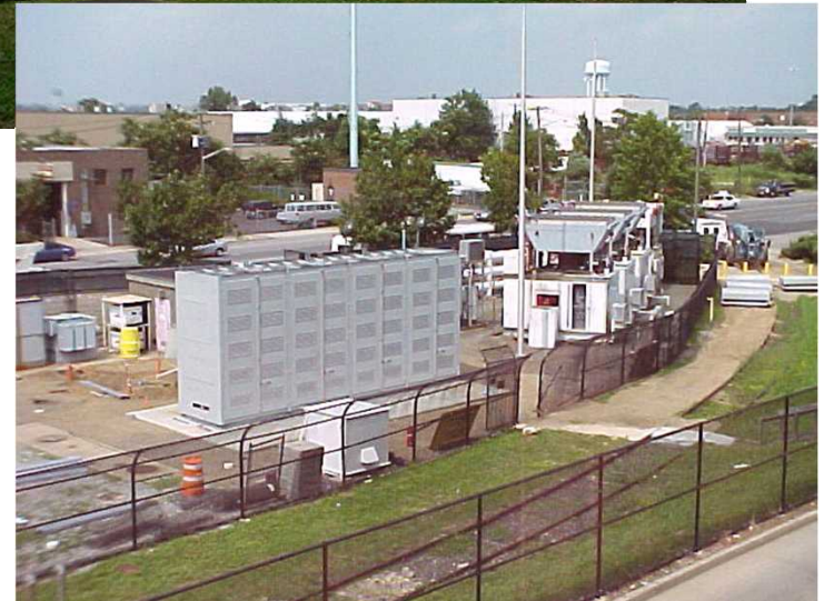
Three 600-HP compressors + 1 MW NaS battery
