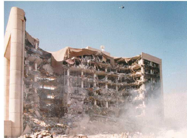
Remains of the Murrah building after blast induced progressive collapse
