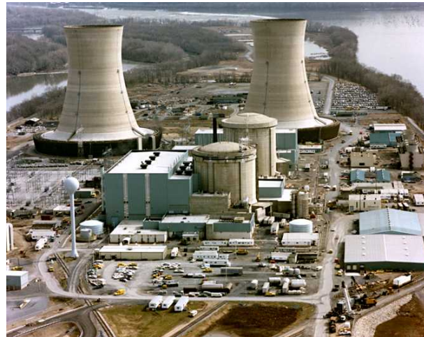
Nuclear Power Plant Cable Insulation
